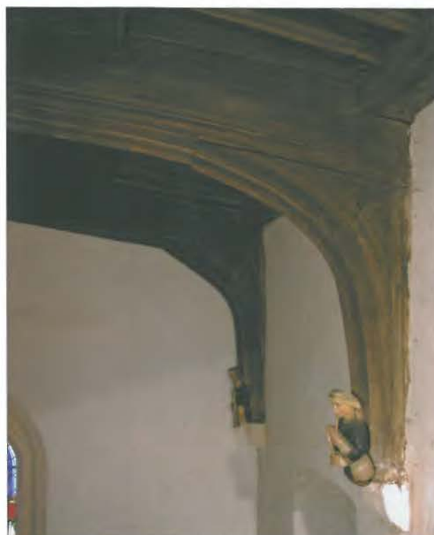
Figs 50, 51, 52: The chancel roof Arch-braces supporting roof beams Purlins and rafters of the chancel roof
