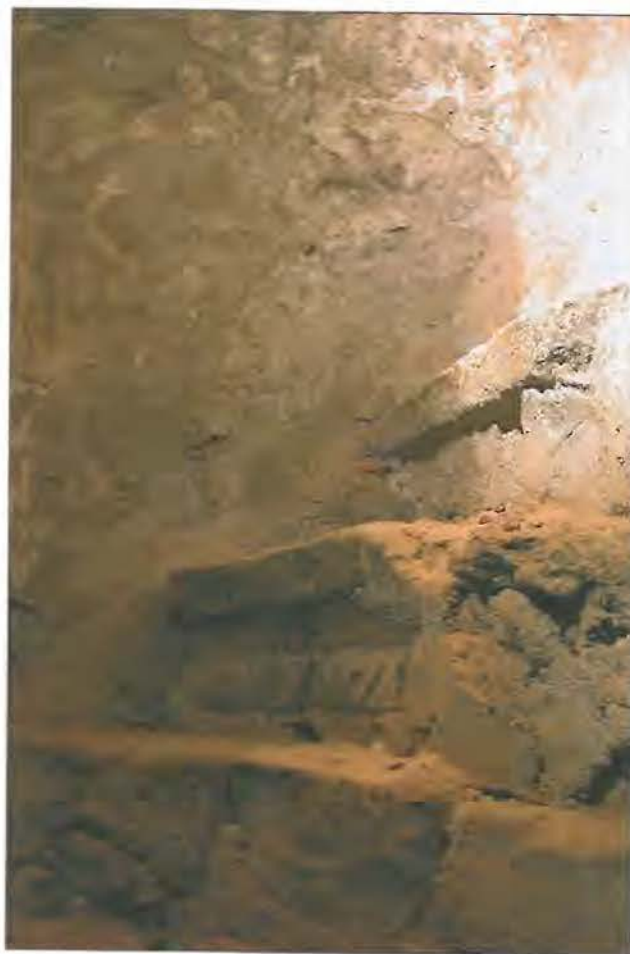
Fig. 23 Tower stair, showing re-used mouldings
