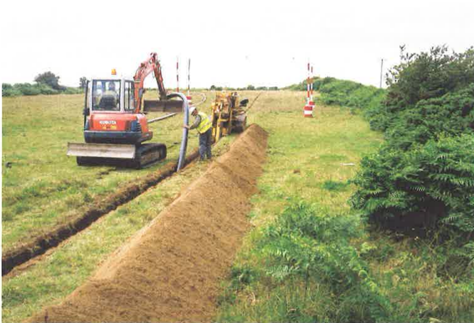
Fig. 17 The pipeline excavation: Trenching through the area of the former medieval strip fields, Feature 20. From the east.
