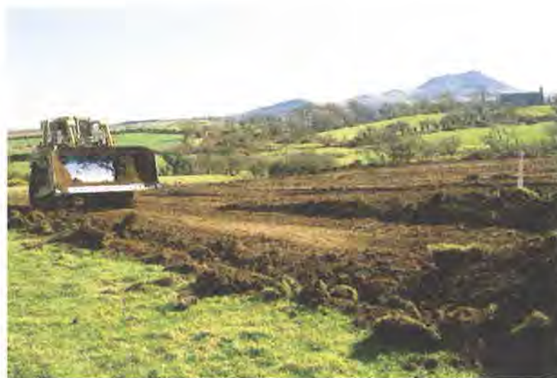
Fig. 3 Machine stripping topsoil: Treatment Works field, Edern
