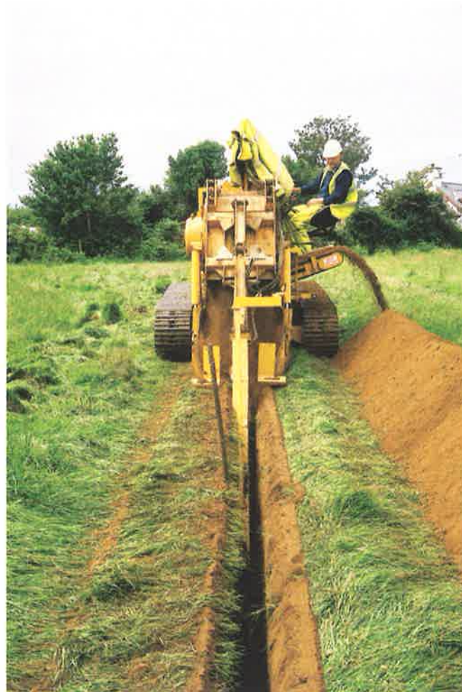
Fig. 15 The pipeline excavation: Mr Griffith's trench cutting machine at work, showing the narrow trench and mechanical soil mixing
