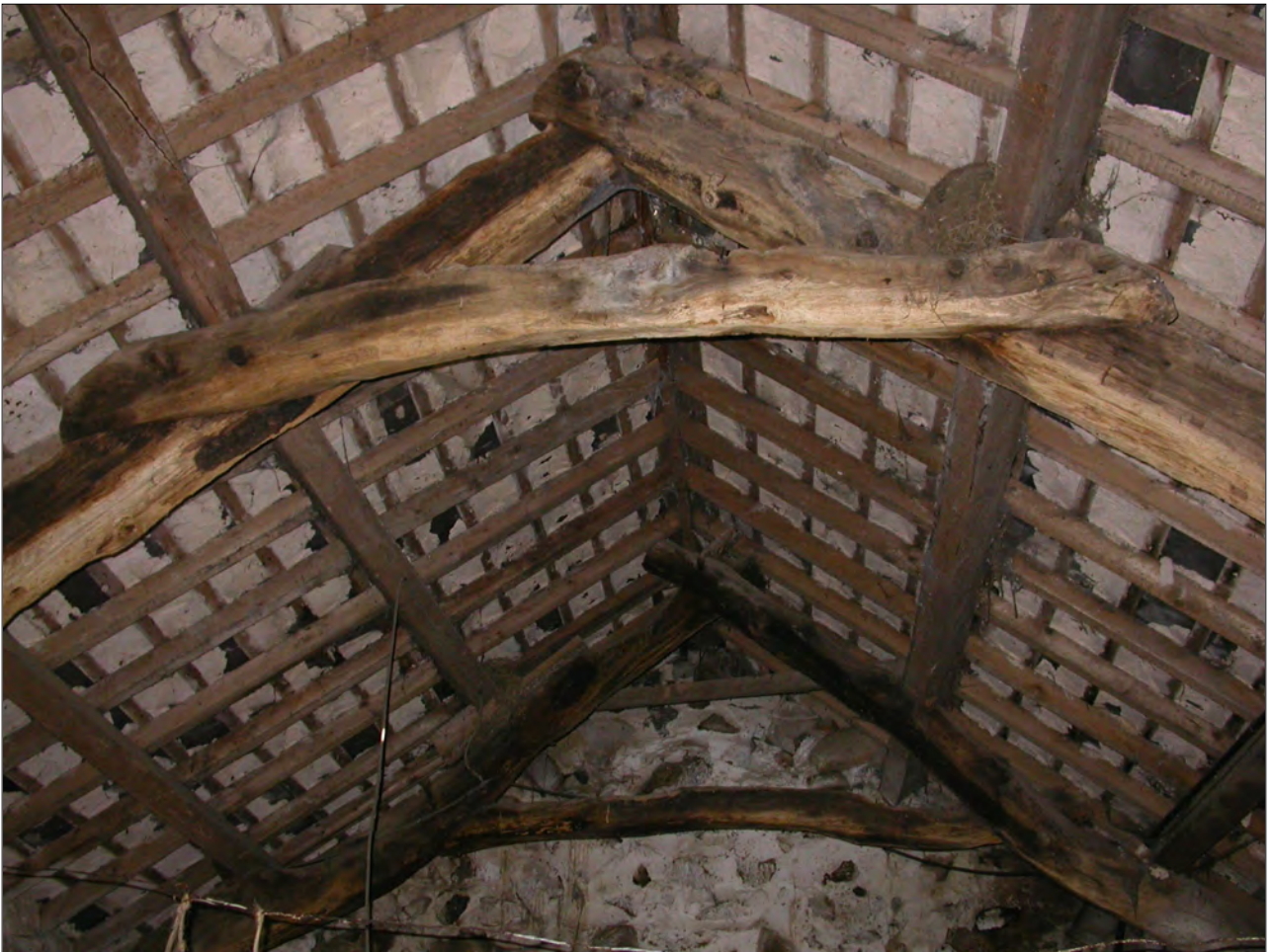
Plate 4. Collar beam roof trusses in structure C
