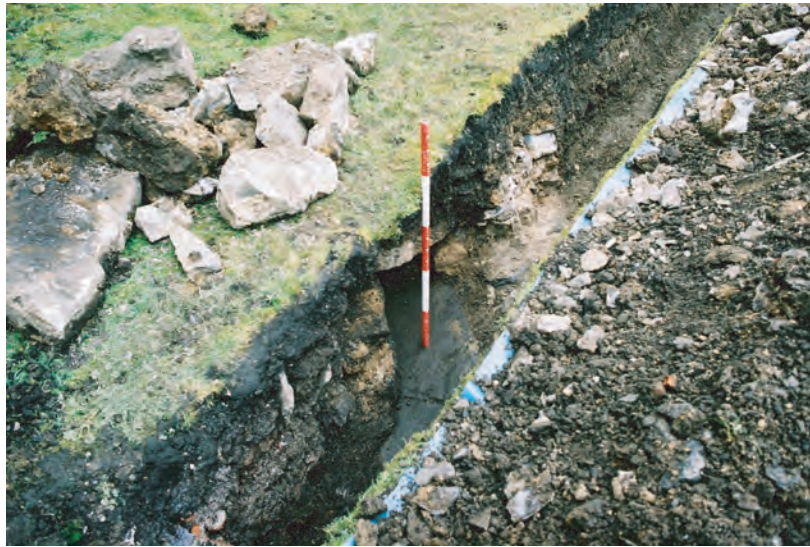
Fig. 9 Beaumaris Gaol: Detail of stone-lined culvert, from the south-east. 1m scale.
