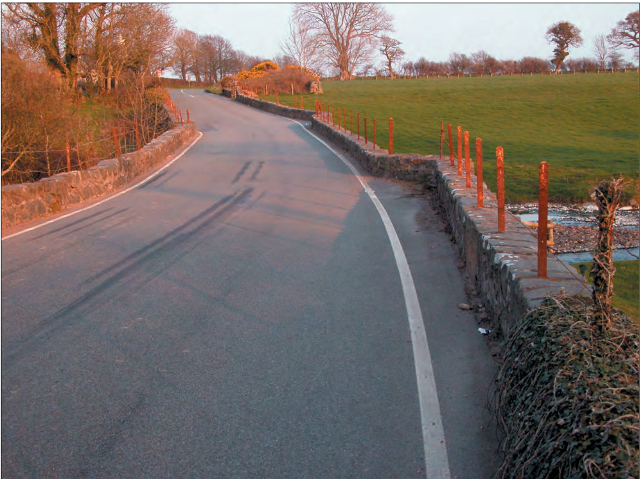
Fig. 5. A497 carriageway looking east, showing road narrowing at bridge and skid marks on carriageway
