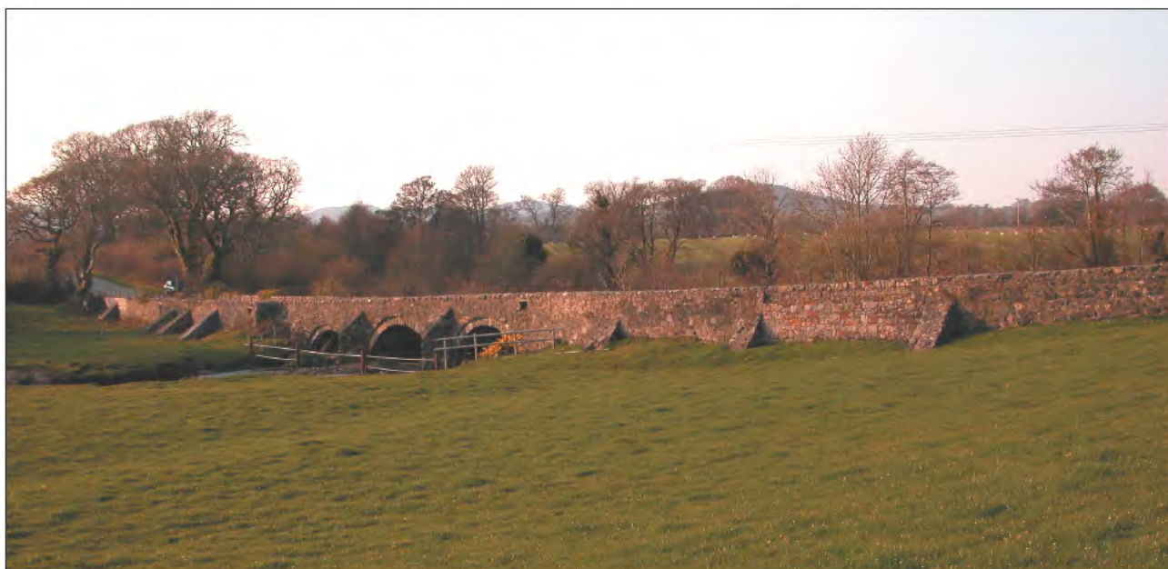
Fig. 3. Pont Bodfel, south side showing bridge, causeways, buttresses and modern repair
