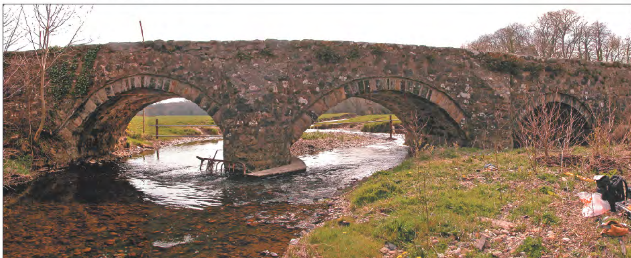
Fig. 3. Pont Bodfel, south side showing bridge, causeways, buttresses and modern repair
