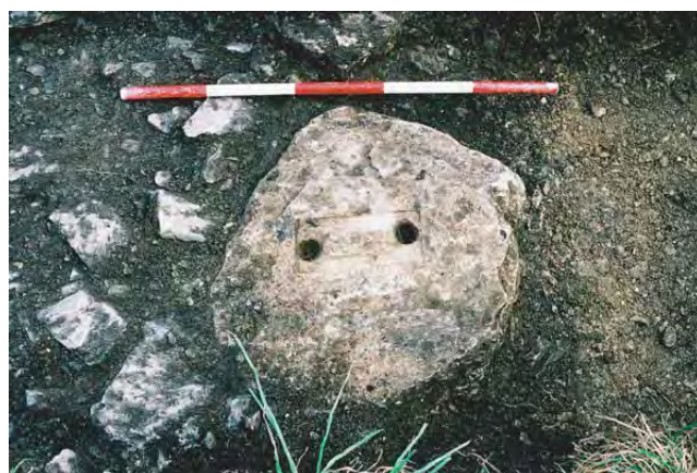
Fig. 8 Hibernia Row Pumping Station Trench 2. Detail of a stone sleeper showing the setting for the iron rail-chair. 1m scale
