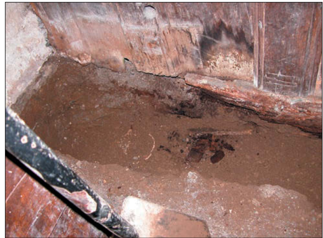
Rotten cill beam at base of screen
