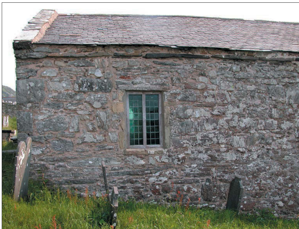
North wall at west end showing re-framed and set chancel window and, immediately to the left of the right hand gravestone, the blocked, early slit window
