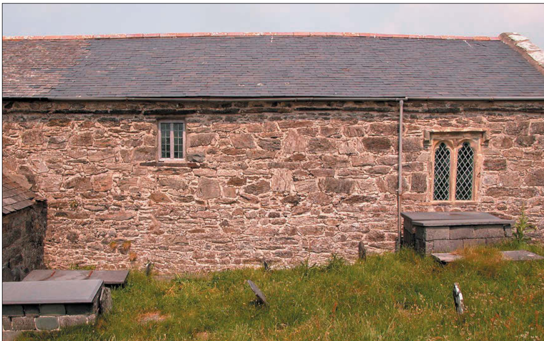
south wall showing masonry phases
