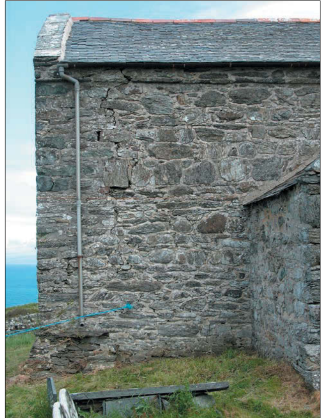
south-west corner showing structural cracks
