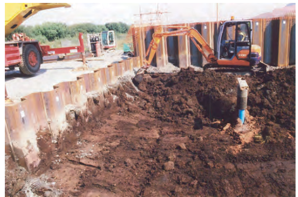
Fairbourne Waste Water Treatment Scheme, Archaeological Watching Brief: Fig. 7 Area B Treatment Works tank construction. Showing clay revealed beneath peat
