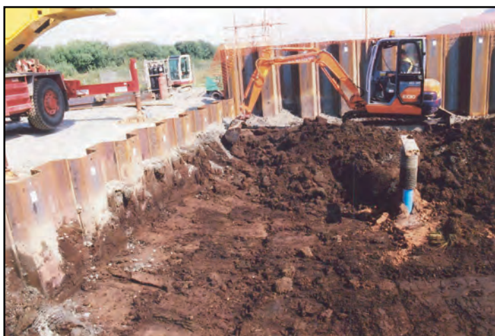
The Treatment Works tank construction, showing estuarine clay revealed beneath the peat and ancient forest horizon
