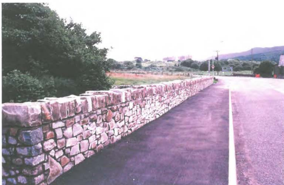
Boundary type 10 - mortared wall
