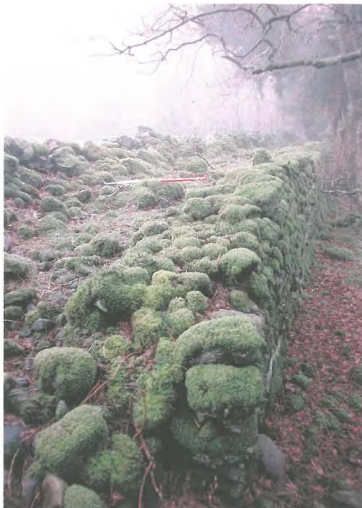
Boundary type 5 - stone-faced drystone wall
