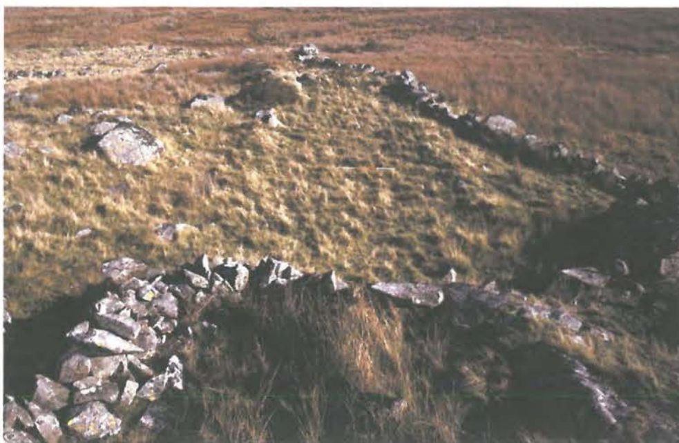
Boundary type 6 - single thickness drystone wall
