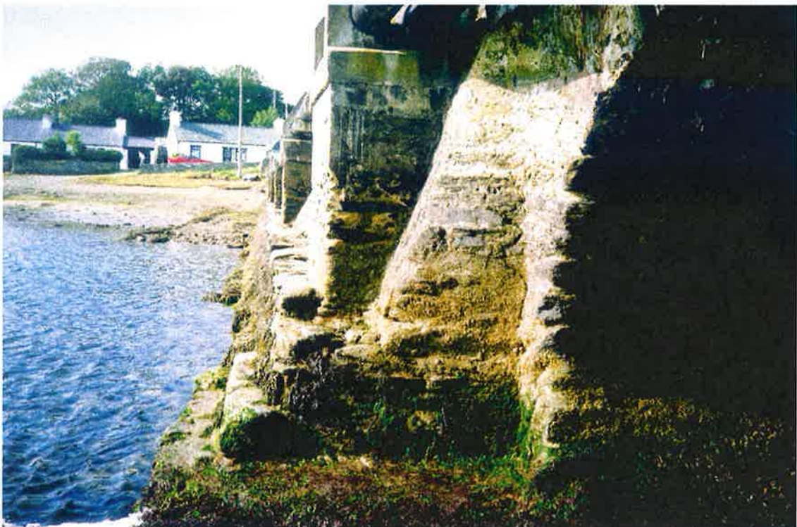
View showing batter, stone base of bridge and stone buttresses
