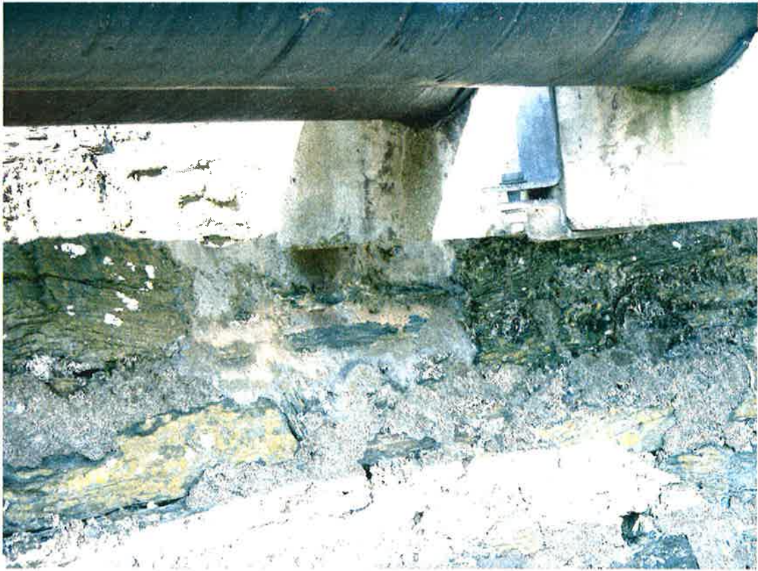
Concrete stanchion inserted into wall
