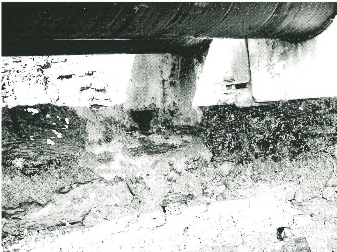
Concrete stanchion inserted into wall
