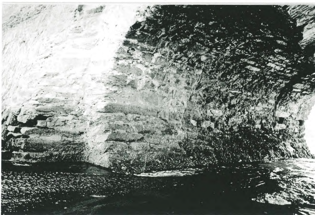
View of east side of culvert
