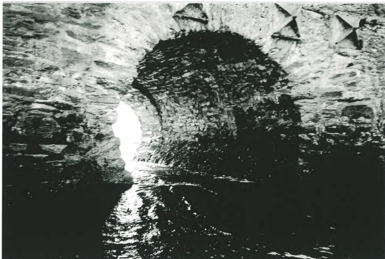
View of west side of culvert
