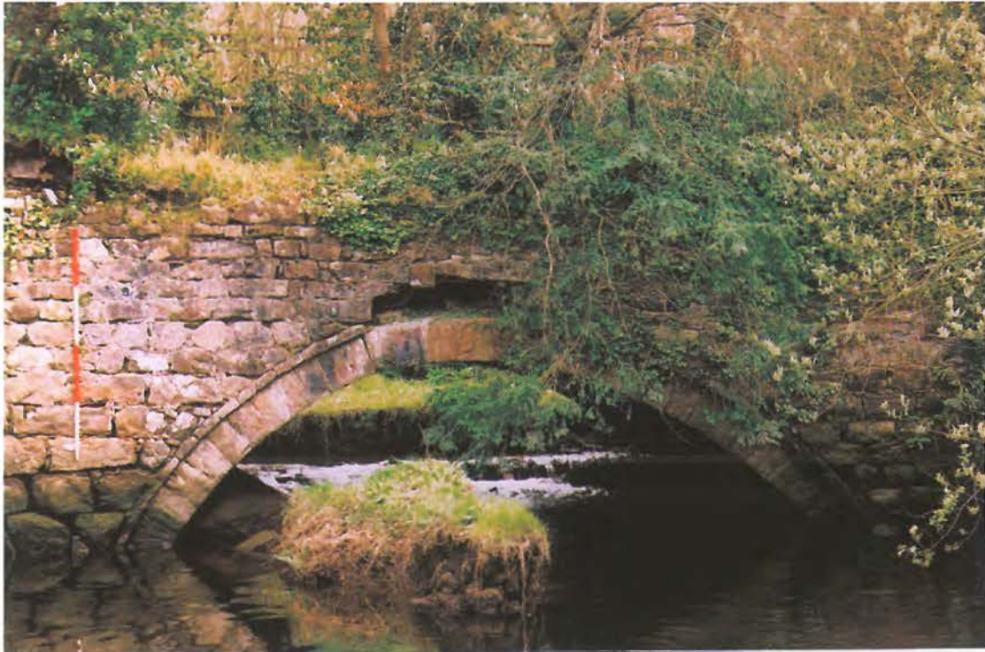
Plate 3 Cegin Viaduct, damage to facing on western side
