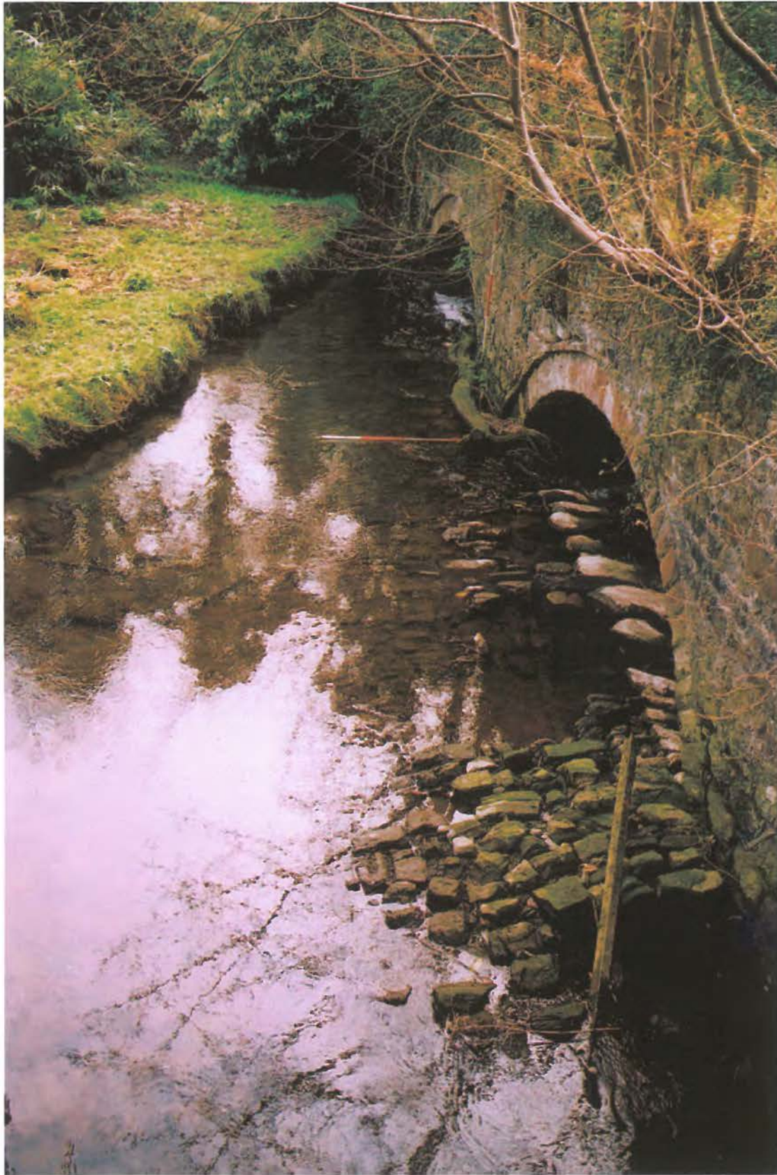
Plate 5 Cegin Viaduct, pitched stone on river bed
