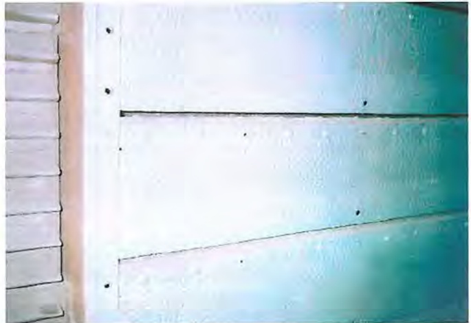
Plate 5 : The sole plates have been removed and the back of the buckets revealed. Here they have been grit blasted and coated with a weldable primer. A combination of rivets and bolts can be seen and the holes through which the sole plates were attached.
