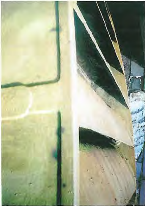
Plate 4 : Pre-restoration view of the original buckets fixed to the internal flanges of the shroud with square headed bolts.
