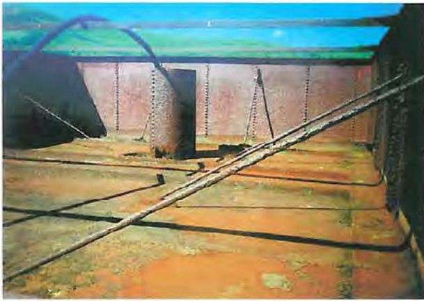
Plate 10 : general view of the header tank before restoration. Note the scaling and the holes in both tank and riser overflow stack.
