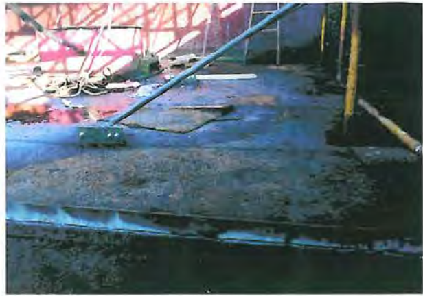
Plate 11 : New upstand, gusseting and internal bracing. Compare with the originals shown in Plate 10. The scaffold is supported on the wall top through holes cut in the tank base and were welded back later.
