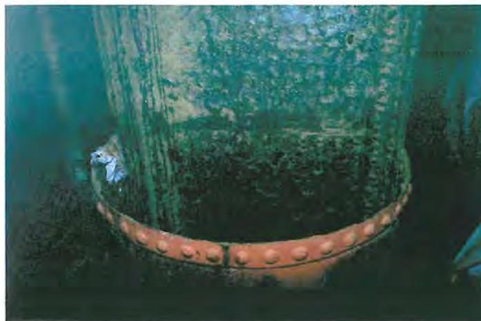
Plate 18 : Where whole new sections were required to be fitted these were welded in inside of the original area so leaving the riveting as original throughout.
