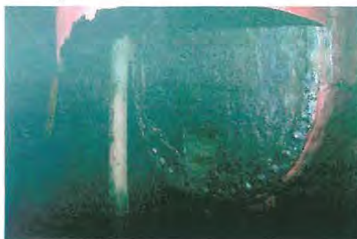
Plate 15 : The mid to lower sections of the riser joined between plates 13,14 and 15. The hand welded seams here are distinguishable by both external cone shaped heads and studs which indicate that the head of the rivet is inside the riser. Note the sections of new metal welded in place.
