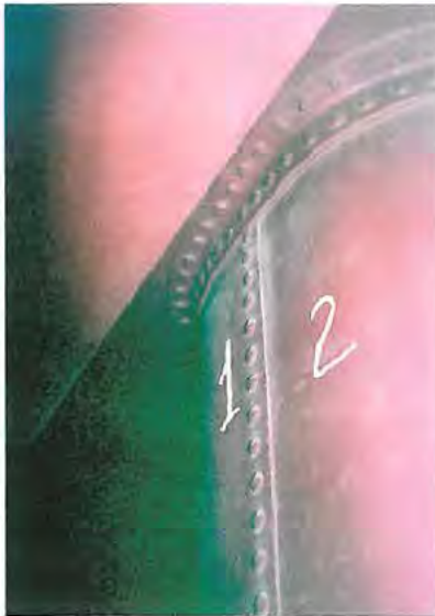
Plate 17 : The uppermost sections of the riser were still in very good condition and after grit blasting and painting appeared as new.
