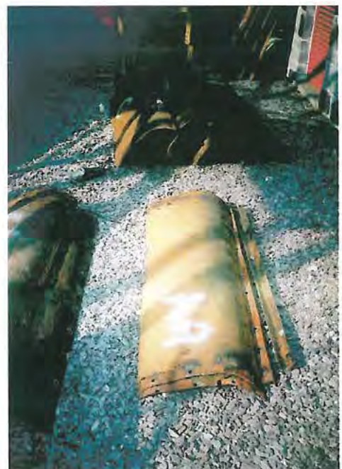
Plate 6 : Sound elements from the most corroded buckets were salvaged for re-use. The buckets were dismantled on site prior to being taken away to be cleaned and incorporated with newly fabricated components.
