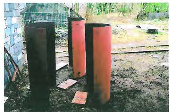
Plate 18 : New sections tailored from dimensions of removed sections used as templates.
