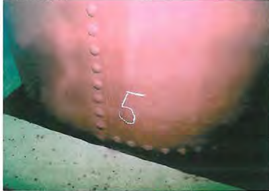
Plate 14 : Hand riveted, staggered seam joining together plate sections 5,6 and 7. Compare the clean dome headed, hydraulically welded seams with the cone shaped hand riveted seams.
