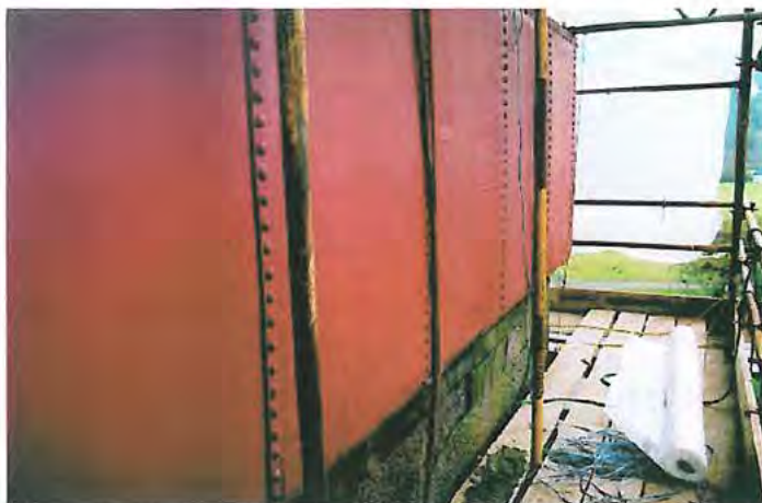
Plate 13 : The external north side of the tank during repairs. New metal has been welded in where necessary and the patches of non-original material left visible as indicated here. Bowling Mill stamp was found on sheet at north-west corner.
