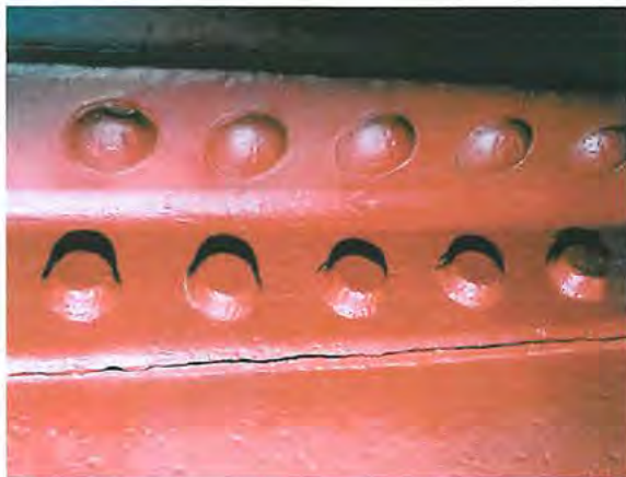
Plate 17 : Revealed on one of the angles connecting the feeder to the header tank - a milling stamp C.C 3
