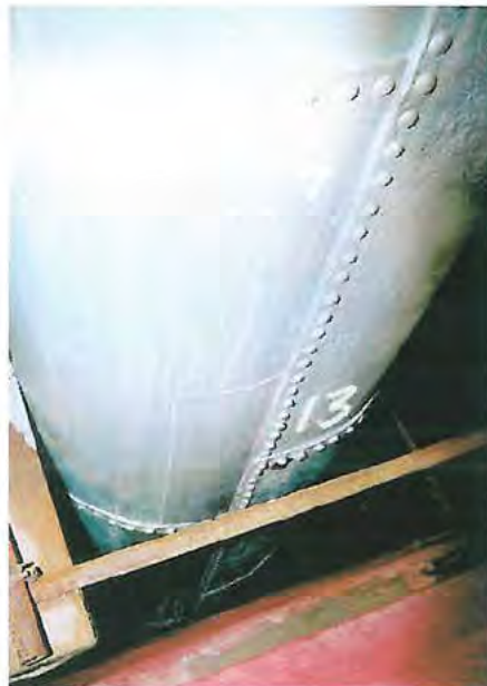
Plate 15 : The mid to lower sections of the riser joined between plates 13,14 and 15. The hand welded seams here are distinguishable by both external cone shaped heads and studs which indicate that the head of the rivet is inside the riser. Note the sections of new metal welded in place.
