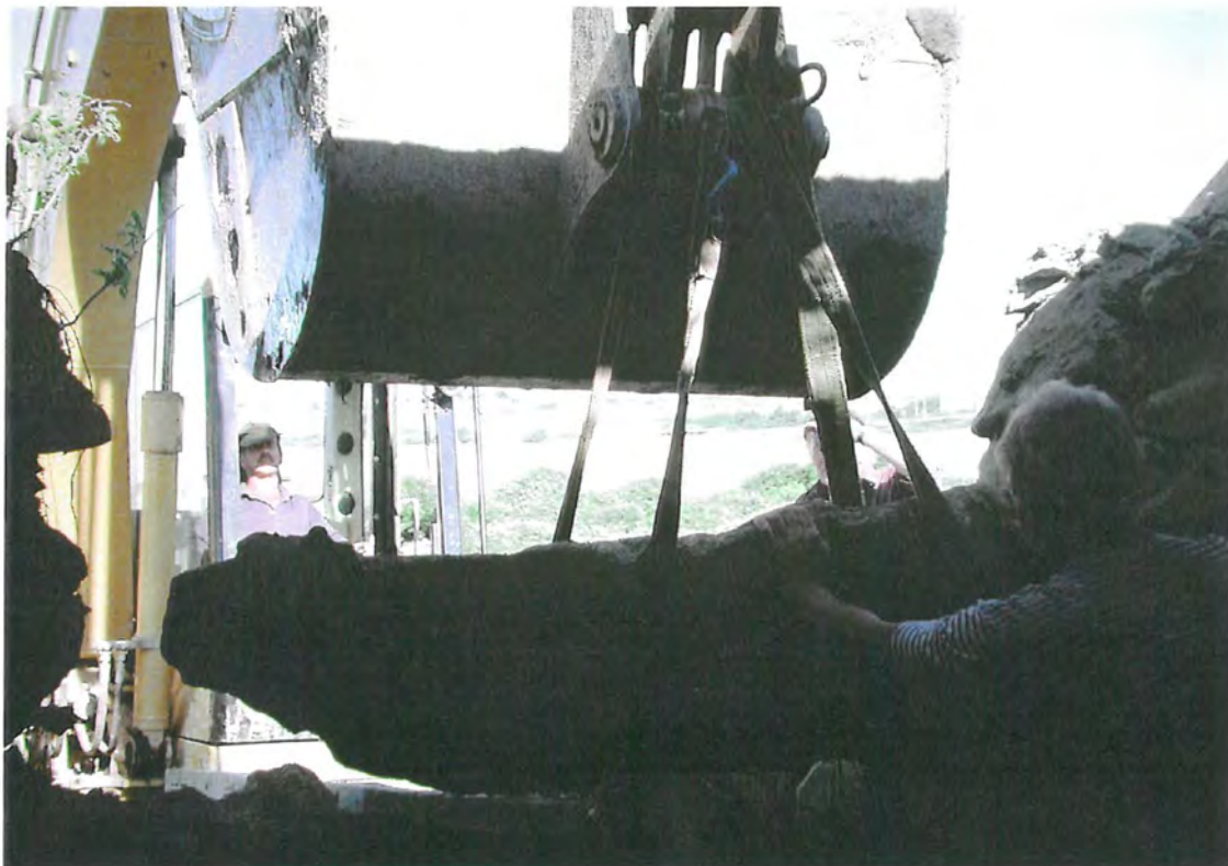
Fig. 5: The hoist is attached and the machine begins to lift the stone
