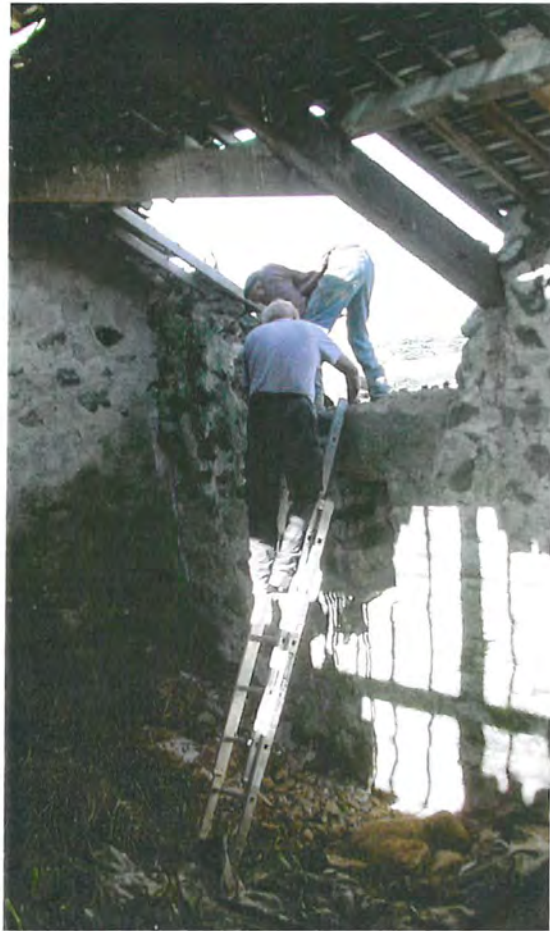
Fig. 4: The stone is exposed in preparation for attaching the hoist
