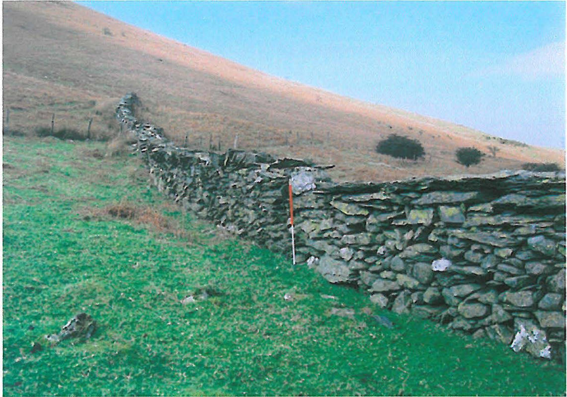
Figure 12 Detail of wall construction style showing overhanging upper courses - PRN 12788
