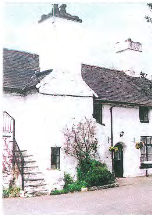
3 Dolgun Uchaf, one of the Quaker houses, is a medieval building with later additions, little changed since the seventeenth century
