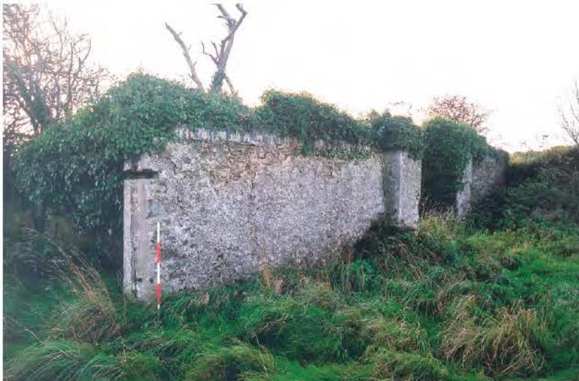
Plate 9: Gateway and farmyard wall at Treddaniel
