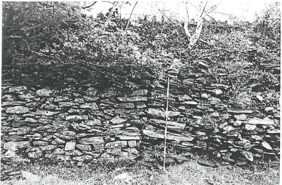
Plate 2: Feature 3, a typical vertical joint
