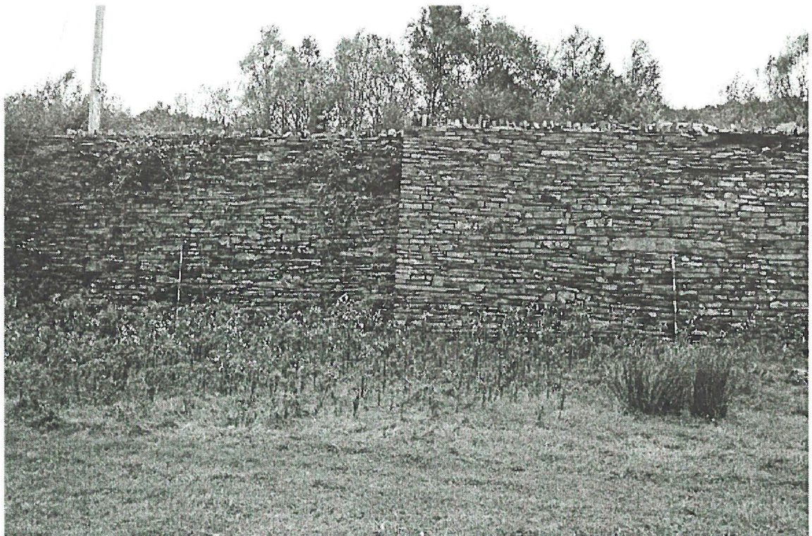
Plate 4: Lay-by buttress
