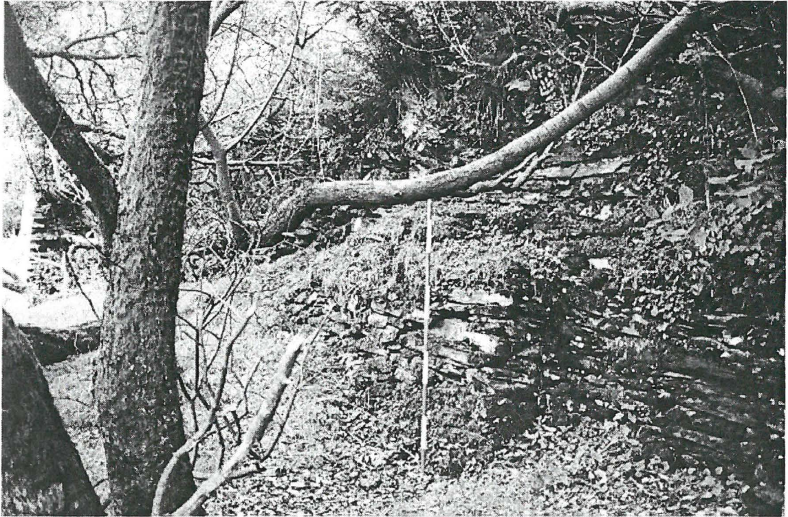
Plate 5: Feature 17, a buttress at the base of the road revetment
