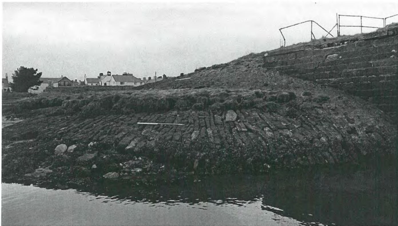
G1578 MALLTRAETH TIDAL DOORS IMPROVEMENT SCHEME NEGATIVE NUMBER: b&w G1578/3/8A SUBJECT: Stone pitching south west of north culvert. Facing north west.
