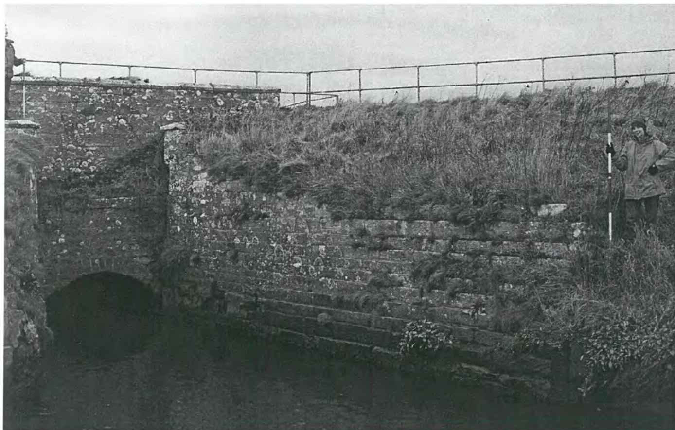
G1578 MALLTRAETH TIDAL DOORS IMPROVEMENT SCHEME NEGATIVE NUMBER: b&w G1578/1/13 SUBJECT: Stepped wing wall, north side of north culvert. Facing south west.
