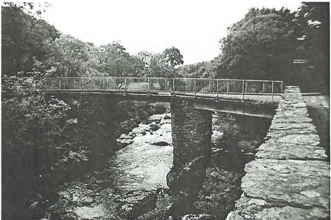
Plate 2. Site 83, Pont-y-Pant, showing rebuilt roadway
