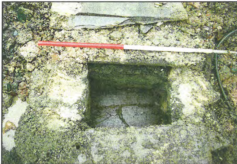
Plate 2: Interior construction of slate-capped culvert
