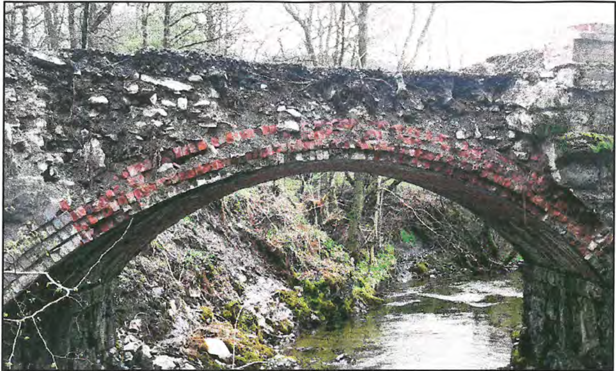
Site 1b - East side of railway bridge during demolition showing construction method
