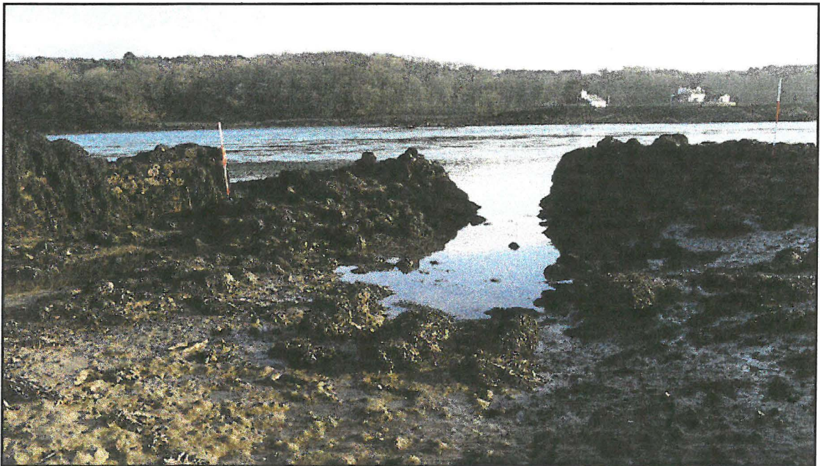
Plate 4: Gorad Ddu - Breach in western wall from NE
