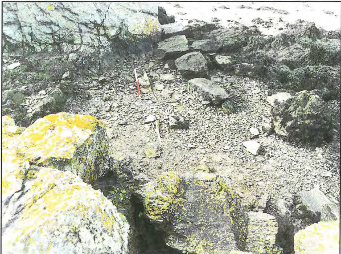
Plate 9 Melin Wen: Mill floor with timber beams
