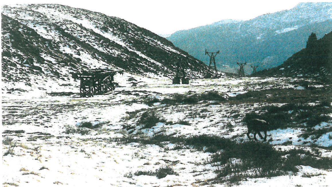
9 Cwm Bychan Mine (PRN: 3792) made use of an aerial ropeway system to carry the ore from the mine itself to a processing area alongside the Welsh Highland Railway.
