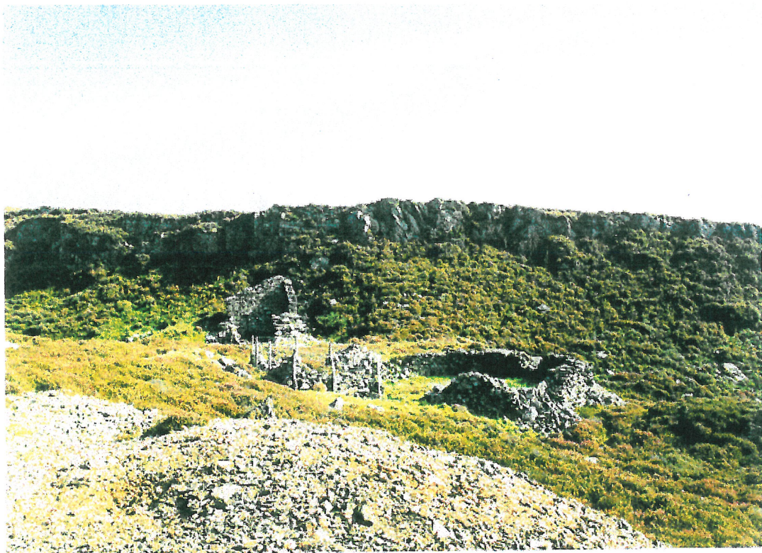
4 This horse-gin circle and steam-engine house illustrate two successive means of raising the ore at Old Clogau Mine. (PRN: 21874)
