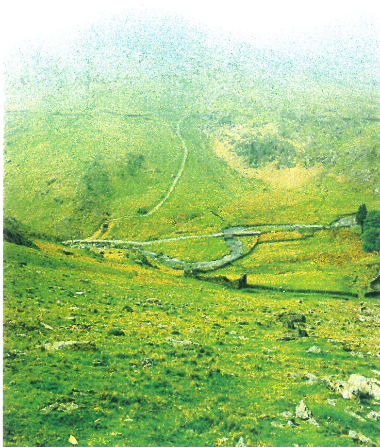
8 Braich yr Oen copper mine (PRN: 21536) is situated on the upper slopes of Yr Arran, south of Snowdon summit, and made use of a complicated variety of transport systems to bring the ore down to the Hafod y Llan mill (PRN: 21156) to be crushed. The course of the lowest stage, a steeply-inclined stone block tramway, is evident here.
