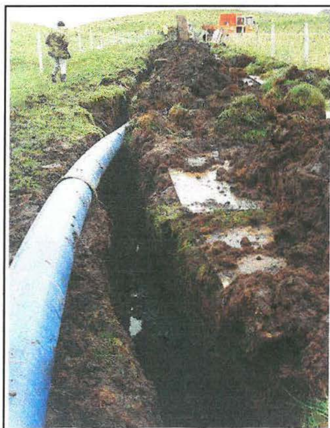
Plate 4 : Excavation through peat west of road
