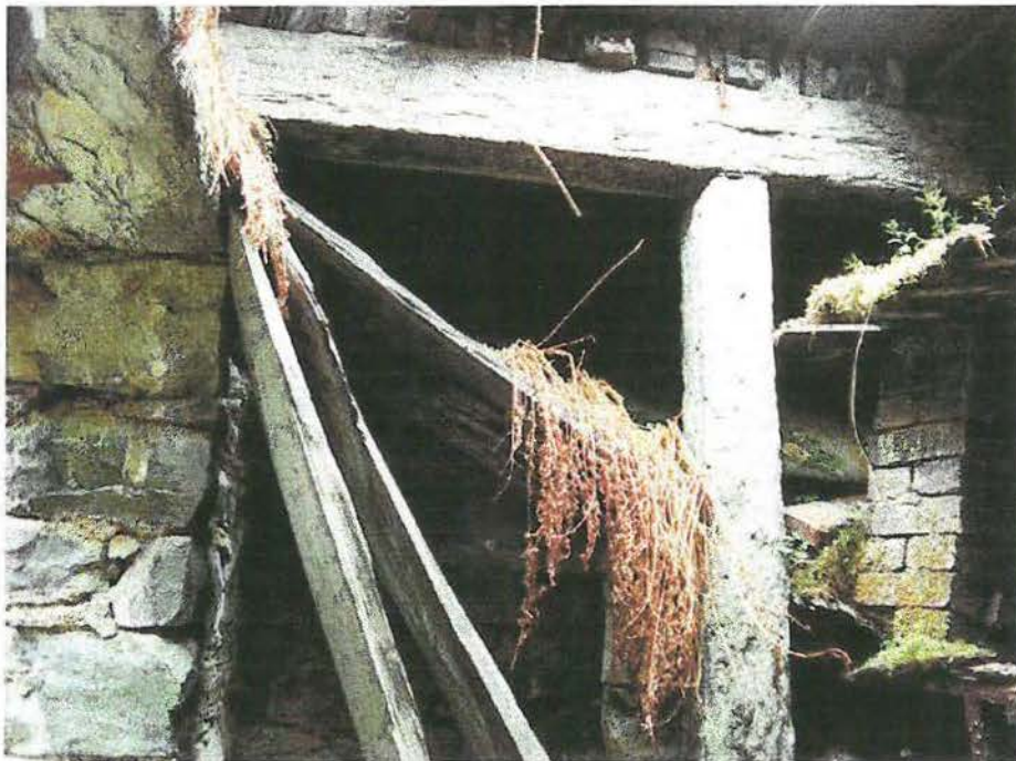
Interior of kiln, showing slate beams and sloping slate slabs
