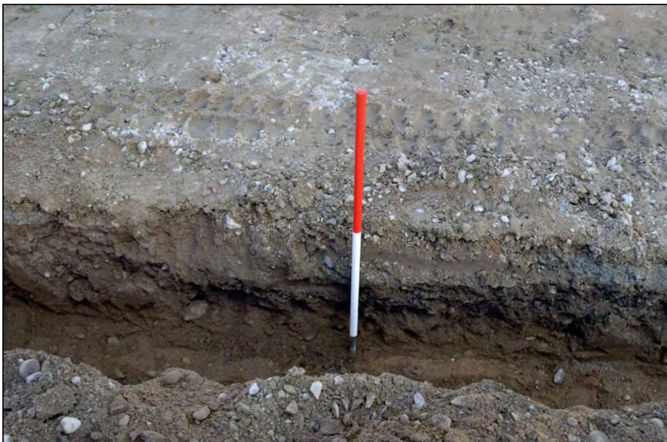
Plate 8: Thin layer of tarmac 0.20m deep in eastern part of the cable trench; scale 1m; view from W (archive reference: G2813_011).
