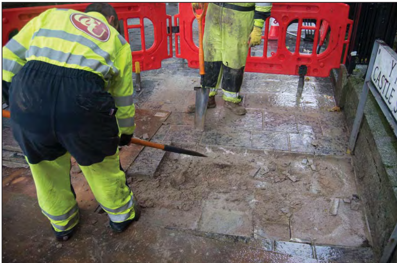
Plate 3: Working shot of removal of concrete mortar mix by hand; scale Not used; view from SW (archive reference: G2798_08).
