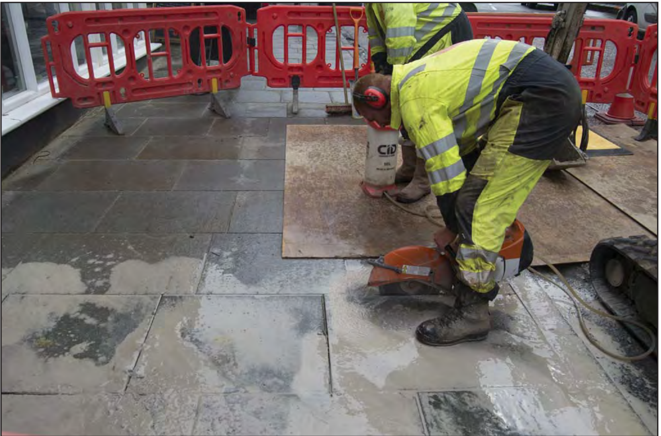
Plate 4: Working shot of work in progress showing cutting of concrete slabs in Trench A using a circular saw - scale not used; view from W (archive reference: G2775_08).
