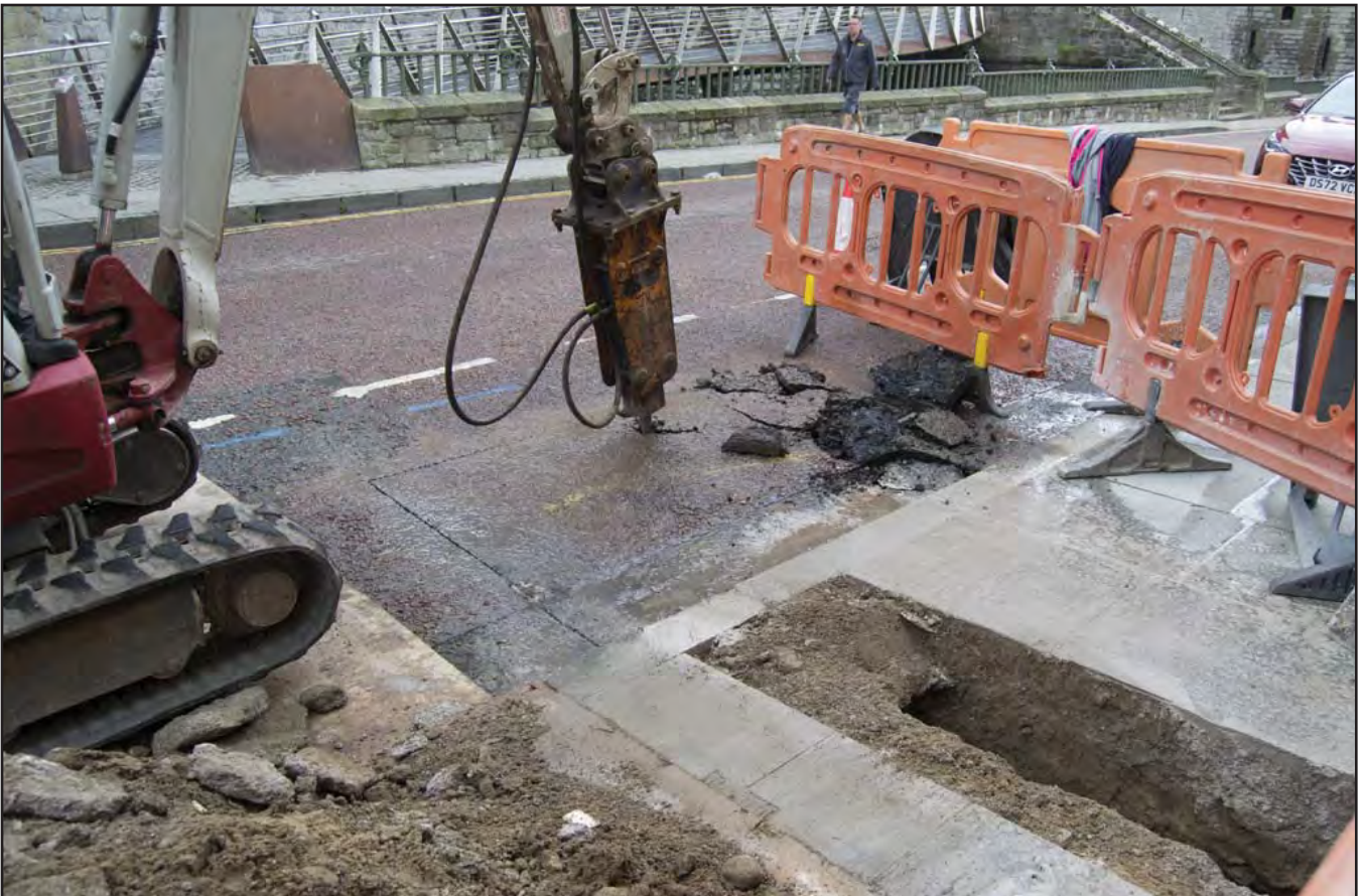
Plate 10: Working shot of road surface broken down by machine as part of Trench B route - scale not used; view from ENE (archive reference: G2775_22).
