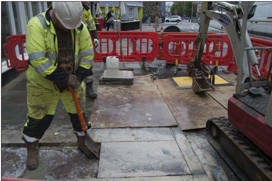
Plate 5: View of removal of concrete pavement slabs in Trench A by shovel and hand - scale not used; view from W (archive reference: G2775_10).
