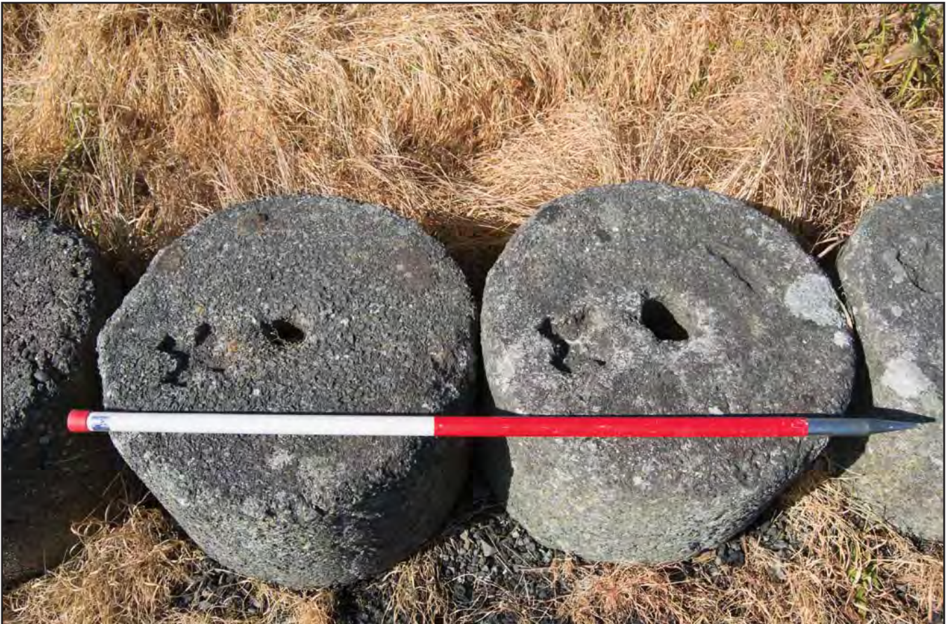
Plate 11: Close-up view of cross indentation/stamp cast atop of several Second World War anti-tank cylinders; view from the south. Scale: 1x1m (archive reference: G2784_009).
