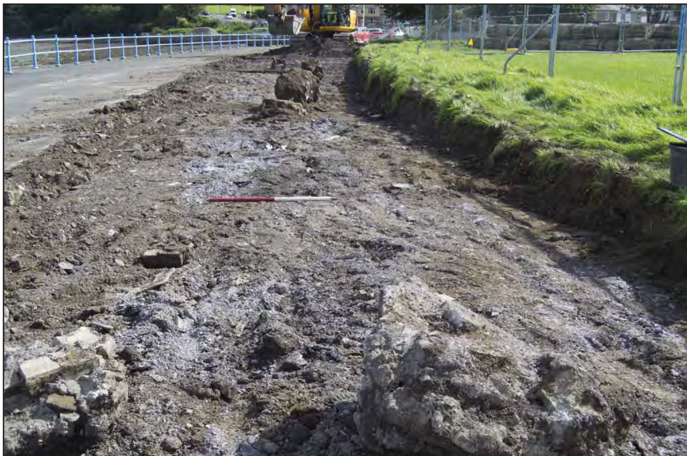
Plate 31: Promenade/King George's playing field after removal of Second World War anti-tank cylinders, showing slate waste and made ground deposits; view from the south-southeast. Scale: 1x1m (archive reference: G2784_143).
