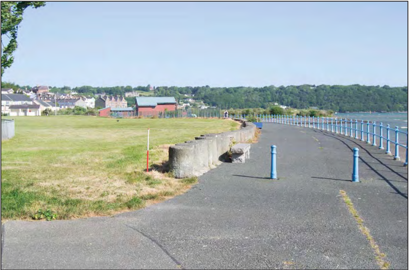
Plate 1: View of cast pebblestone concrete Second World War anti-tank cylinders along promenade; view from the south-southeast. Scale: 1x1m (archive reference: G2784_001).
