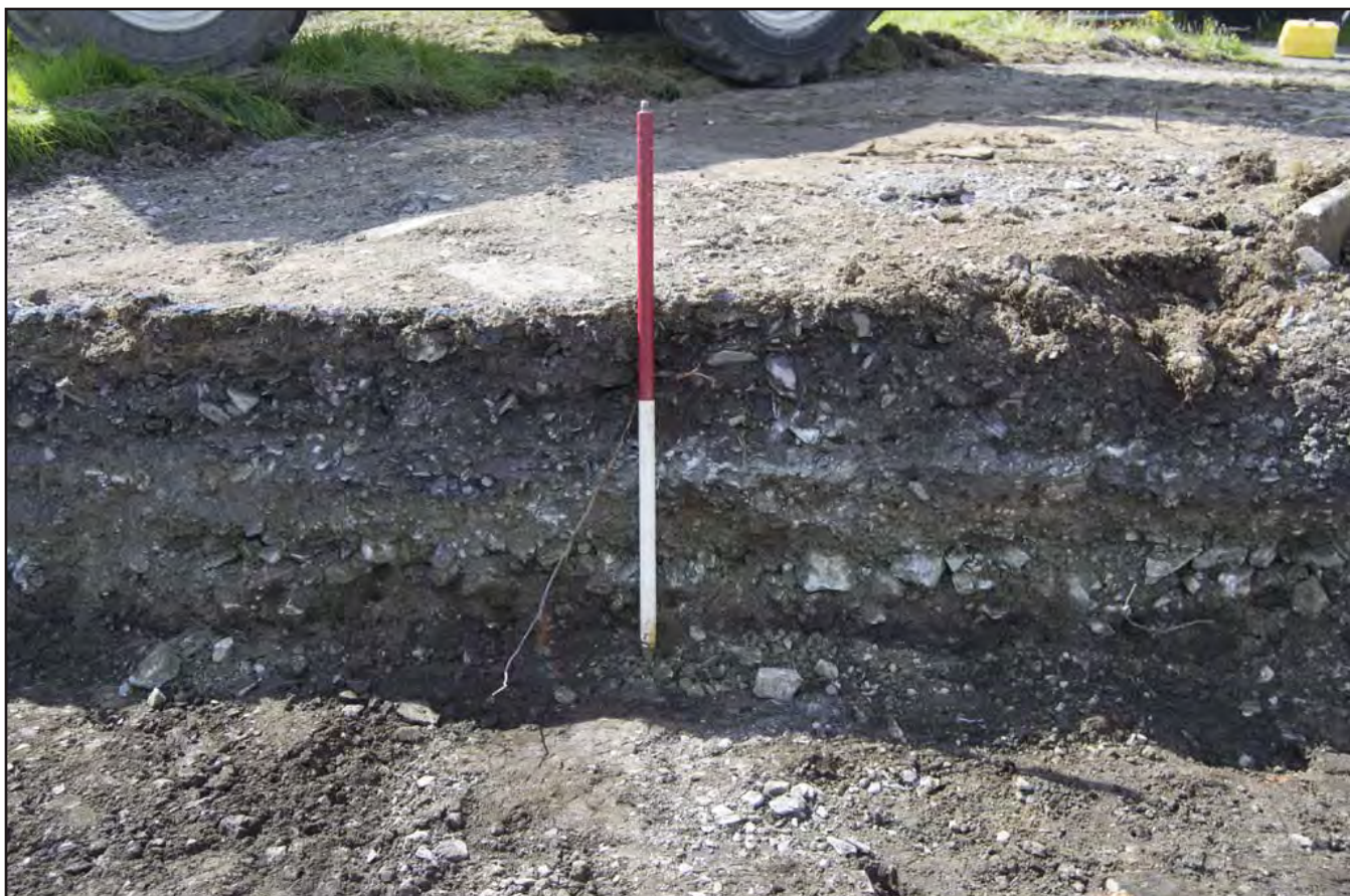
Plate 24: Northeast facing section of haul road excavation showing made ground. Scale: 1x1m (archive reference: G2784_061).
