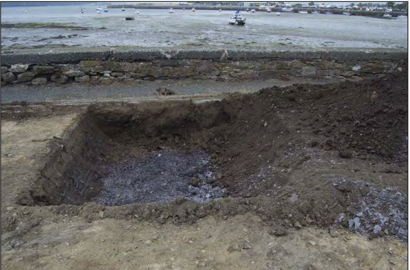
Plate18: Small trial pit within the recreational area on completion of the topsoil strip showing crushed slate, likely used to create a level area; view from the southwest (archive reference: G2784_039)
