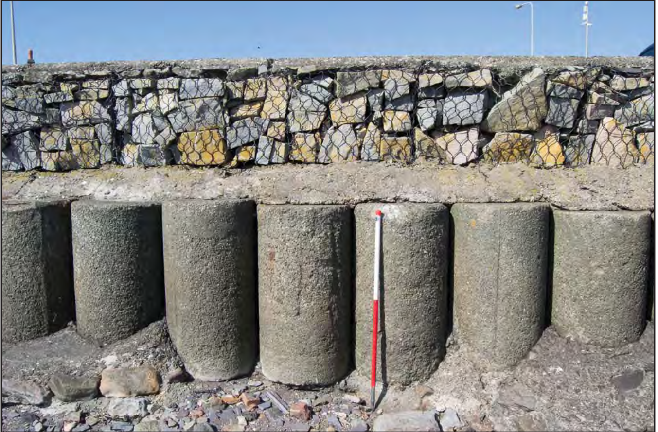
Plate 7: Close-up view of Second World War anti-tank cylinders reused within the coastal defence wall, along with stone filled gabion baskets; view from the east-northeast. Scale: 1 x1m (archive reference: G2784_019).
