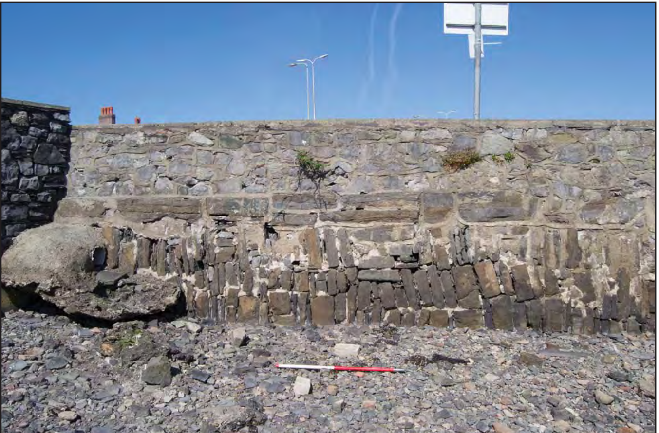
Plate 14: Close-up view of stone phasing within the coastal defence wall below the recreational area and next to the slipway; view from the east-southeast. Scale: 1x1m (archive reference: G2784_023).
