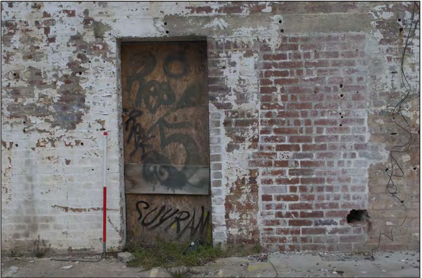
Plate 7: A2 Unit - View of phasing of blocked up doorway into A6; scale 1x1m; view from E (archive reference: G2756_07).
