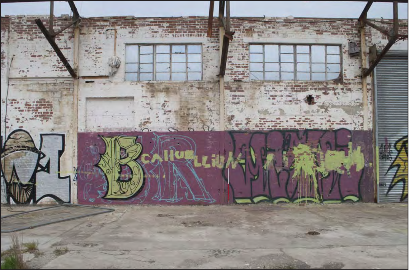
Plate 10: A2 Unit - View of blocked up former garage doorways and window; scale 1x1m; view from E (archive reference: G2756_10).
