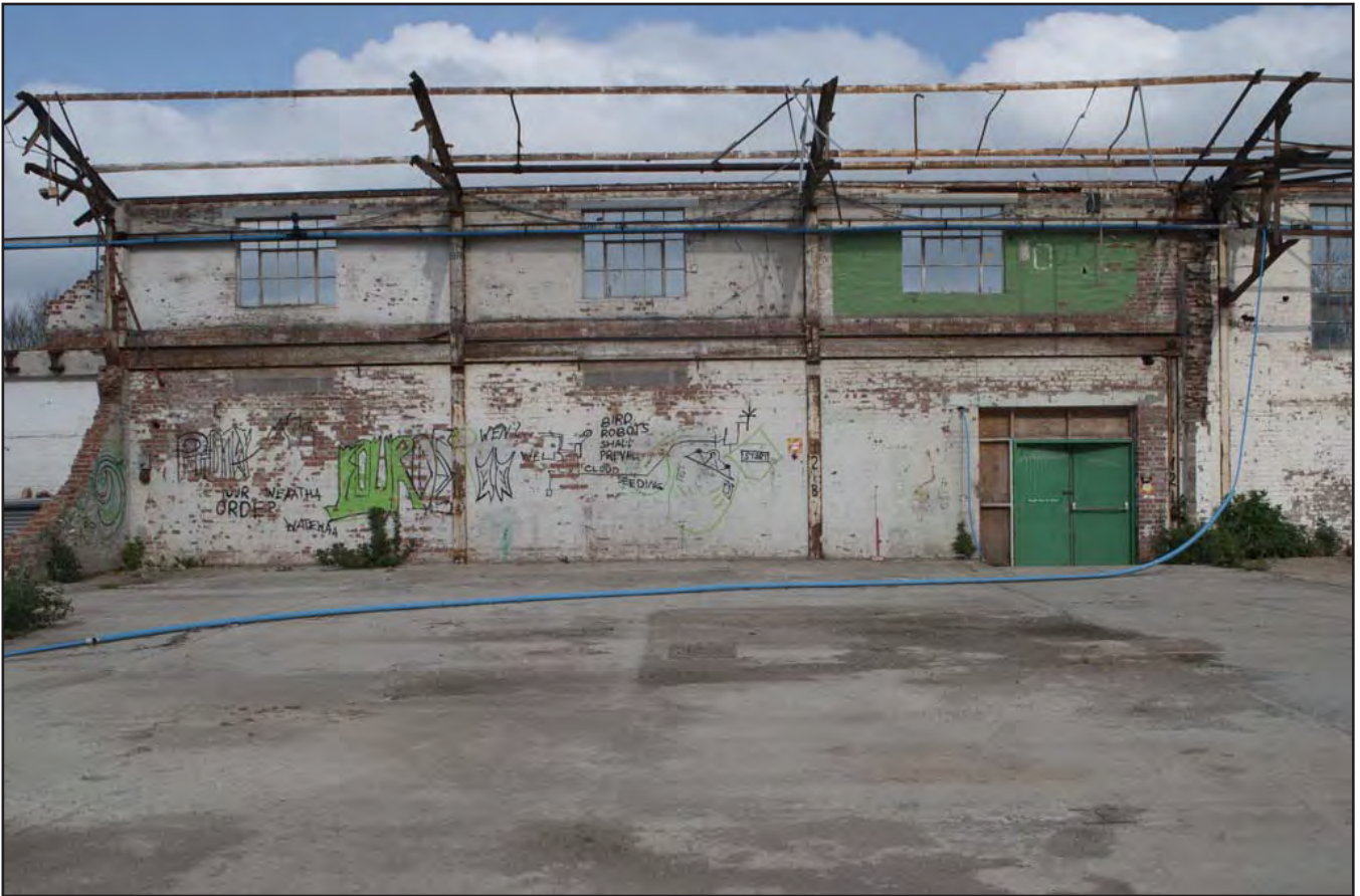
Plate 5: A2 Unit - View of south end interior of A2 showing steel casement windows and former garage entrance; scale 1x1m; view from SE (archive reference: G2756_05).
