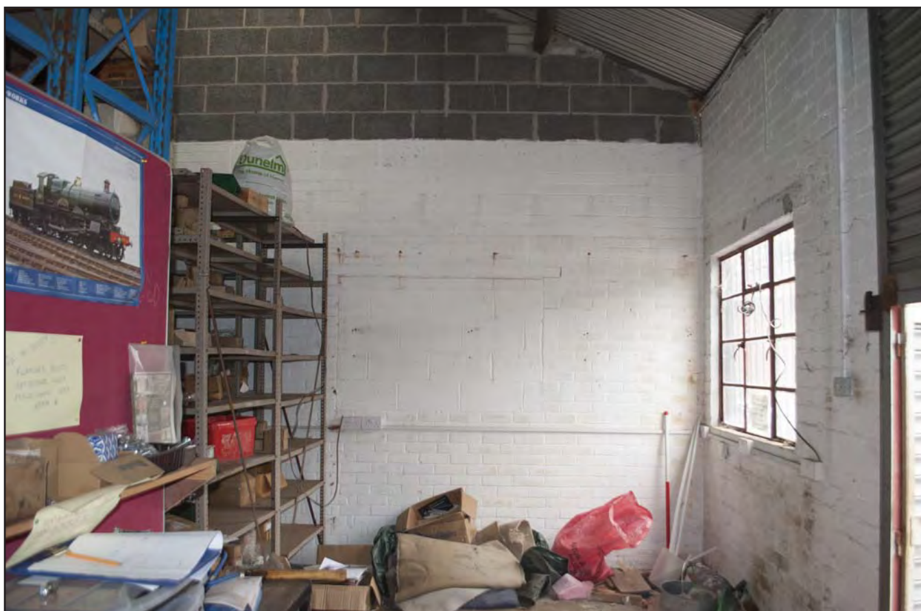
Plate 86: Interior G2 - View of blocked up window in G2 and breeze block partition; scale 1x1m; view from S (archive reference: G2756_100).
