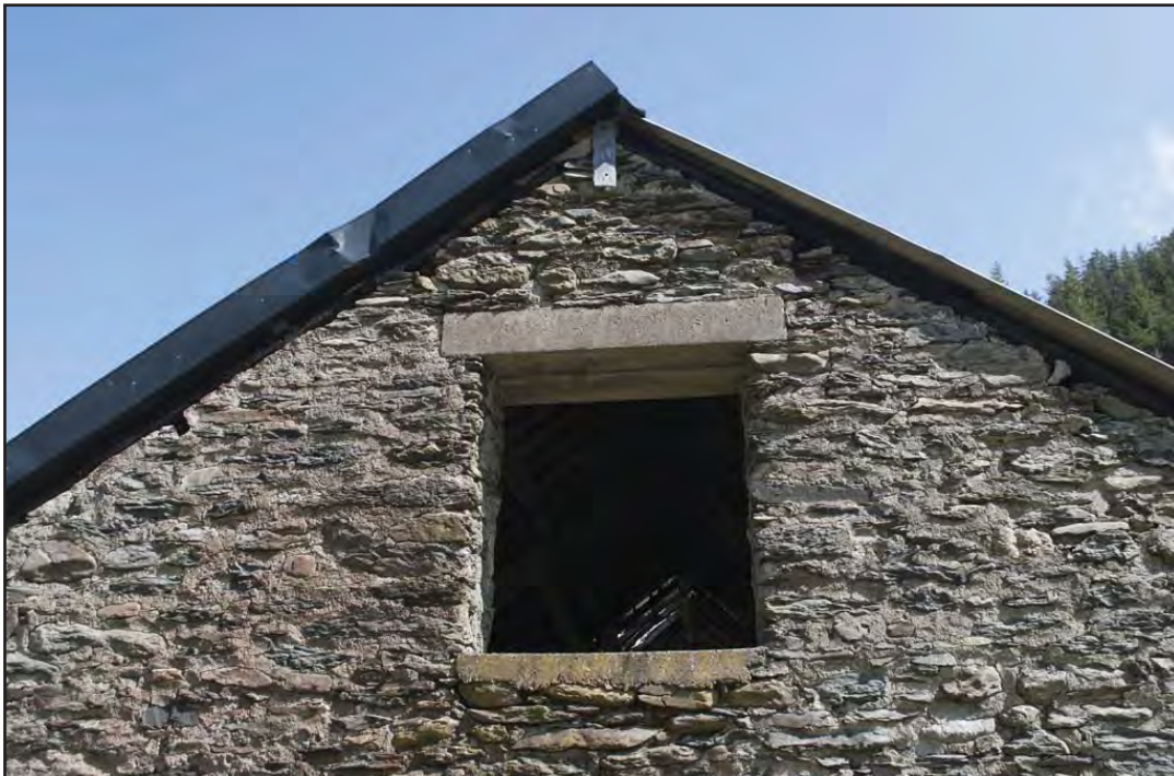
Plate 14: Exterior - Close-up of window with concrete lintels and roof of barn; scale not used; view from S (archive reference: G2778_014).
