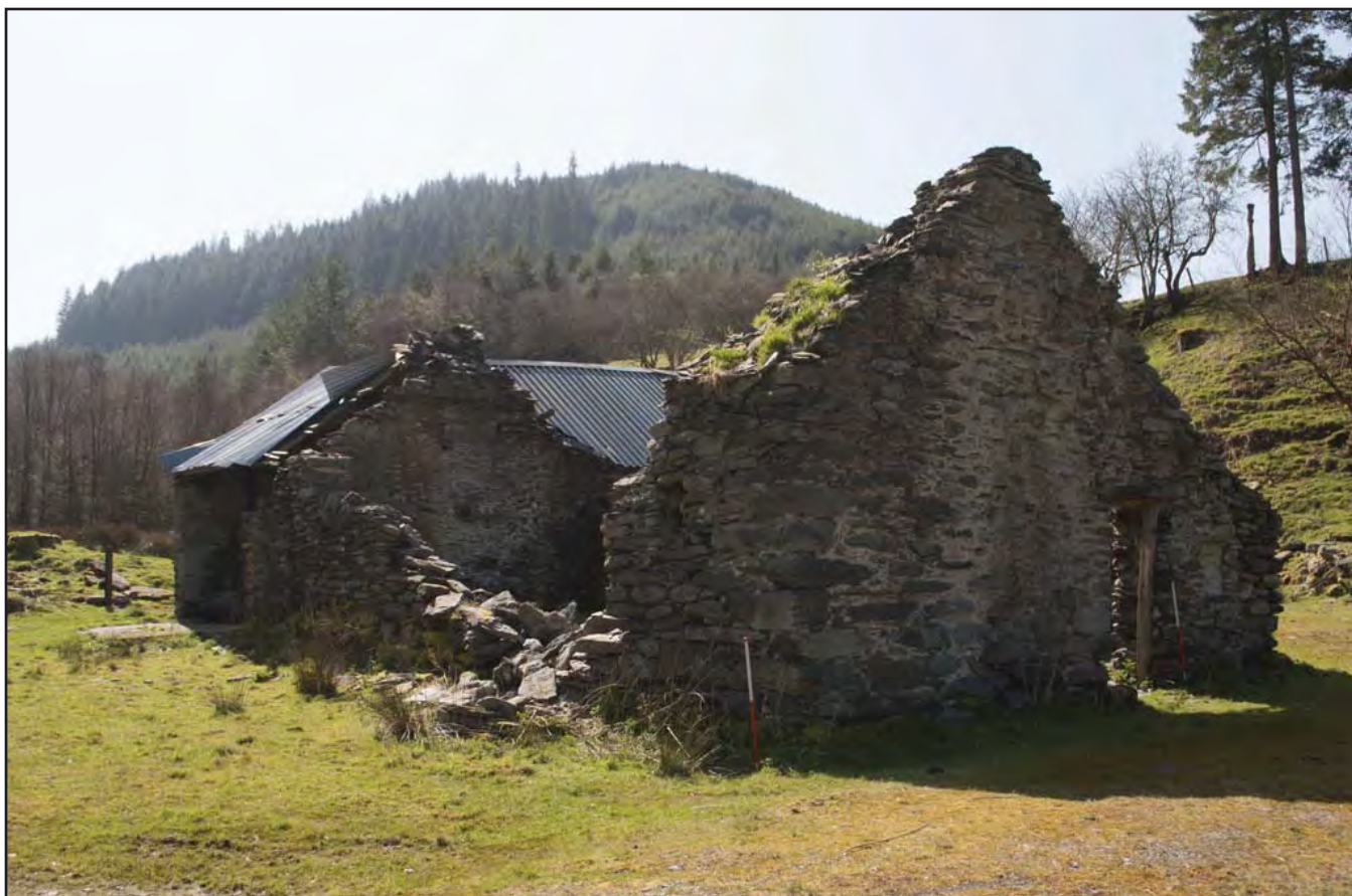
Plate 8: Exterior - Oblique view of N corner of cottage showing collapsed wall; scale 2x1m; view from N (archive reference: G2778_008).
