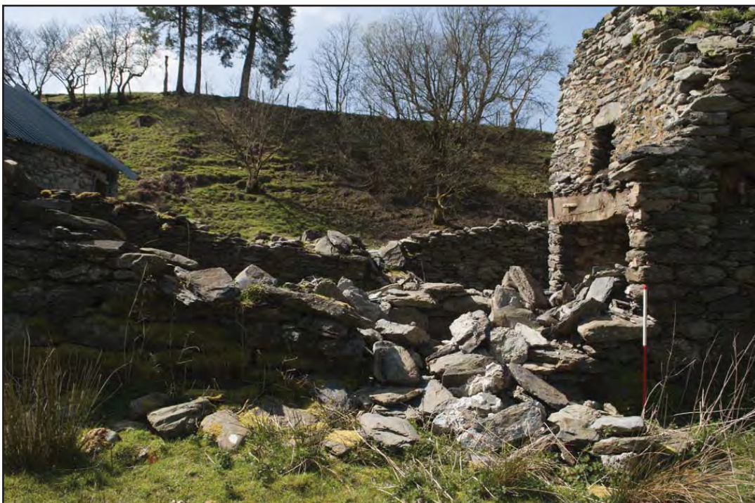
Plate 20: Exterior - View of collapsed NE wall of cottage and fireplace within; scale 1x1m; view from NE (archive reference: G2778_020).
