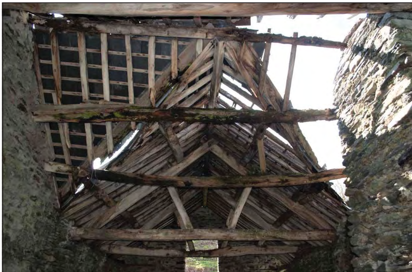
Plate 30: Interior Barn - View of trussed roof inside barn showing collapse; scale not used; view from E (archive reference: G2778_030).
