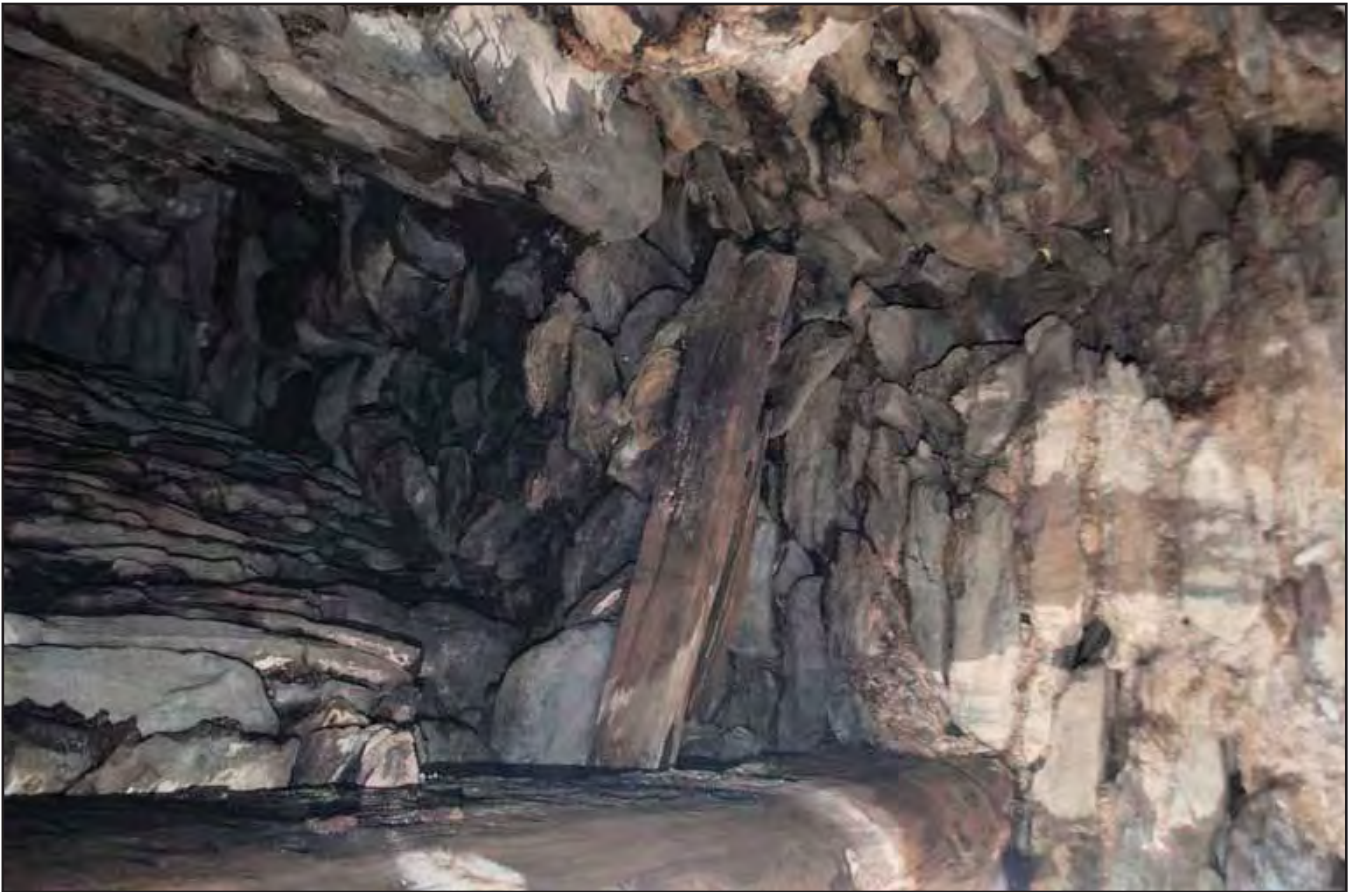
Plate 53: Interior Cottage - View up into fireplace chimney in cottage, showing collapsing beam; scale not used; view from E (archive reference: G2778_053).
