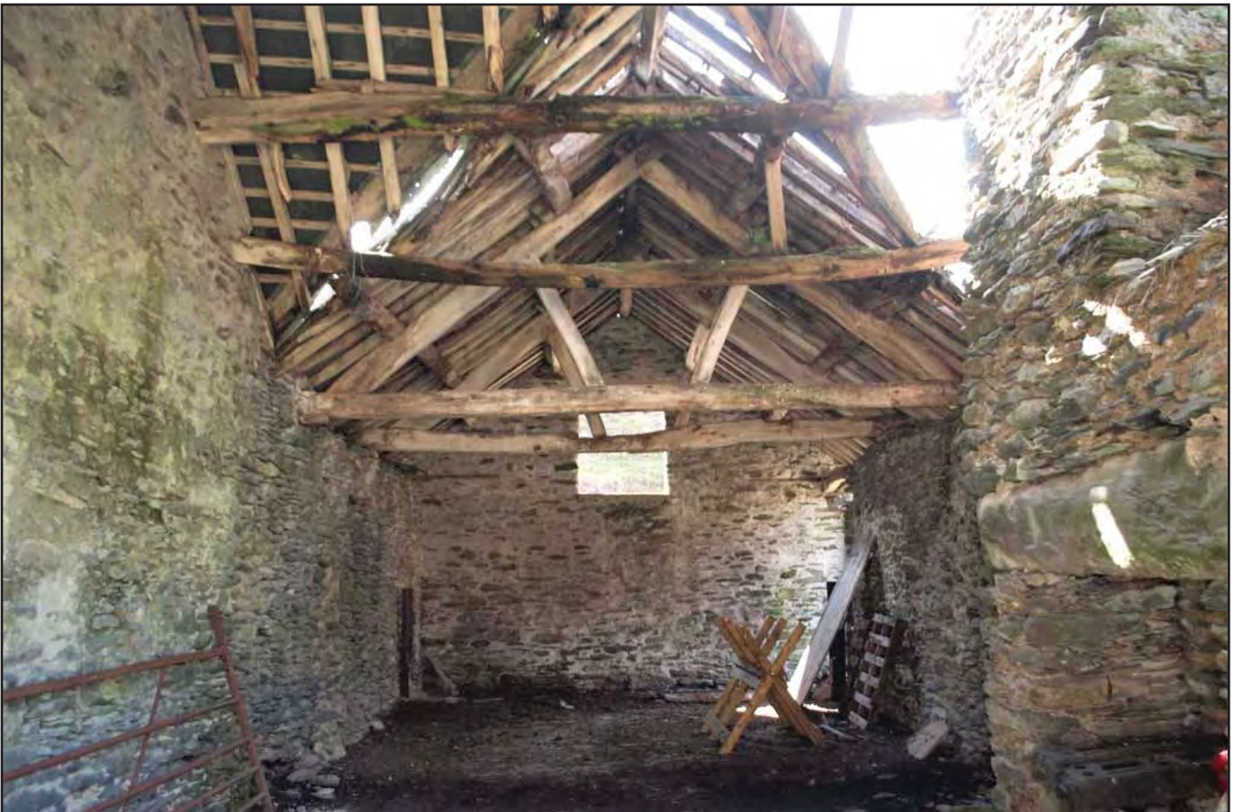
Plate 34: Interior Barn - View into barn from large entrance showing roof trusses; scale not used; view from E (archive reference: G2778_034).
