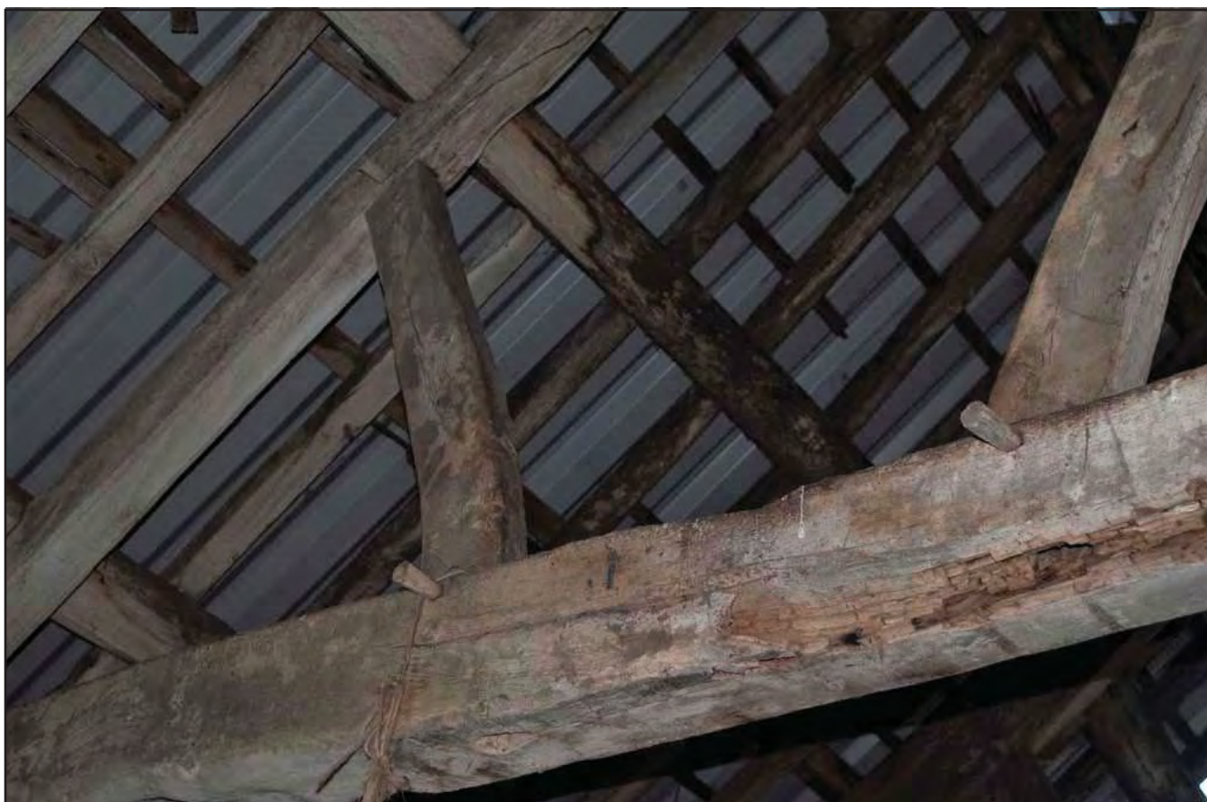
Plate 32: Interior Barn - Close-up of wooden pegs in trussed roof; scale not used; view from SW (archive reference: G2778_032).
