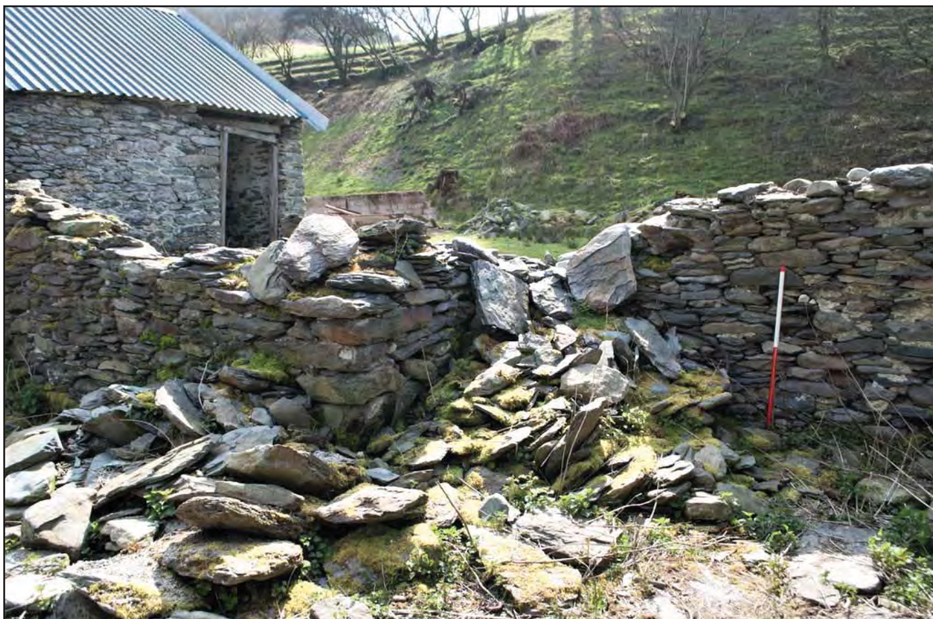
Plate 48: Interior Cottage - View of SW wall of the cottage showing collapse; scale 1x1m; view from N (archive reference: G2778_048).
