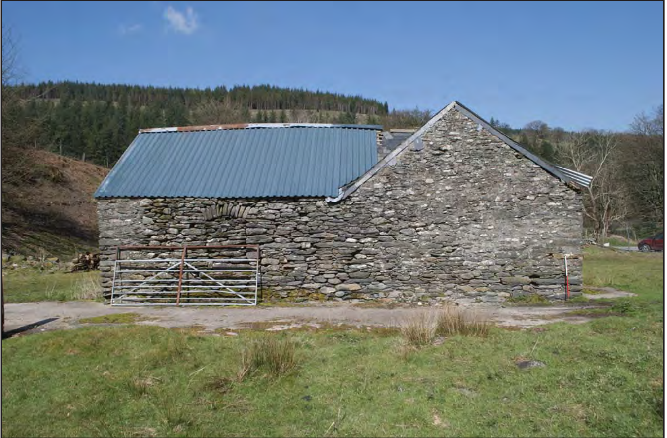
Plate 3: Exterior - View of exterior SE wall of barn, showing window infilled with stone; scale 1x1m; view from SE (archive reference: G2778_003).
