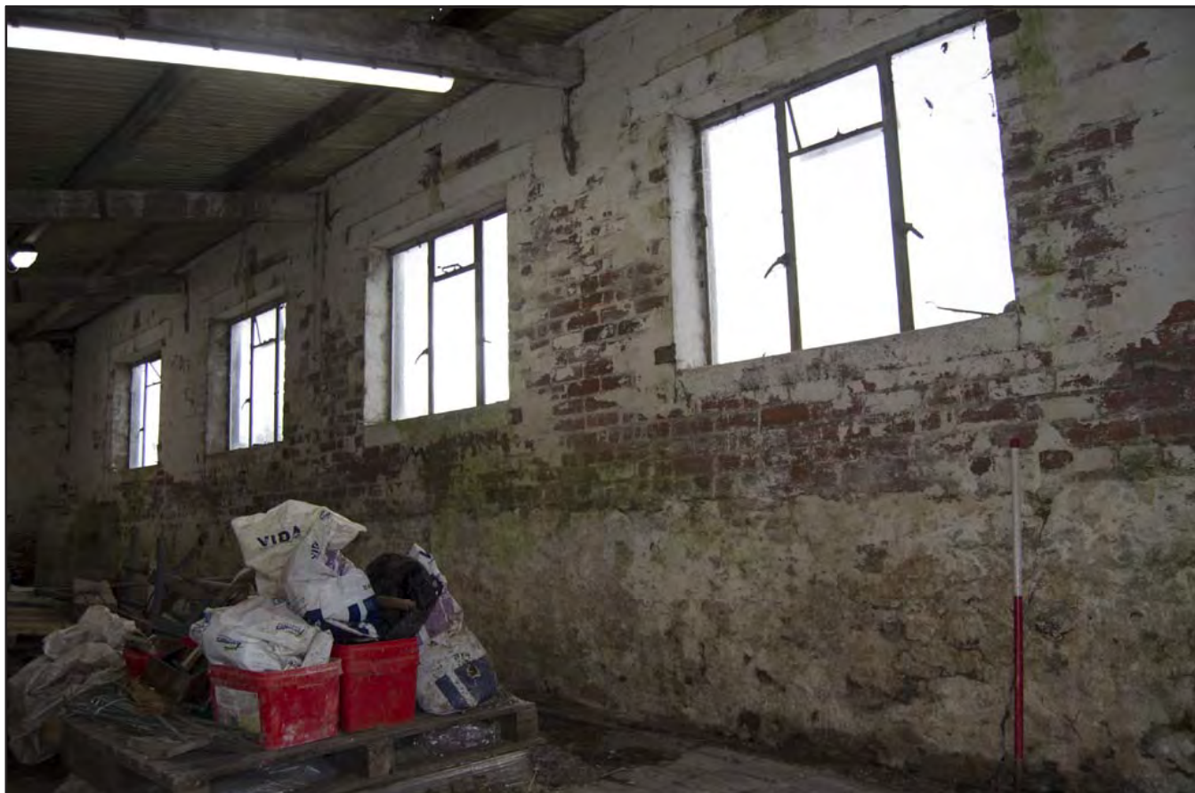
Plate 15: Room 1 - View of steel casement windows within brickwork at SW edge of Room 1; scale 1m; view from N (archive reference: G2743_15).
