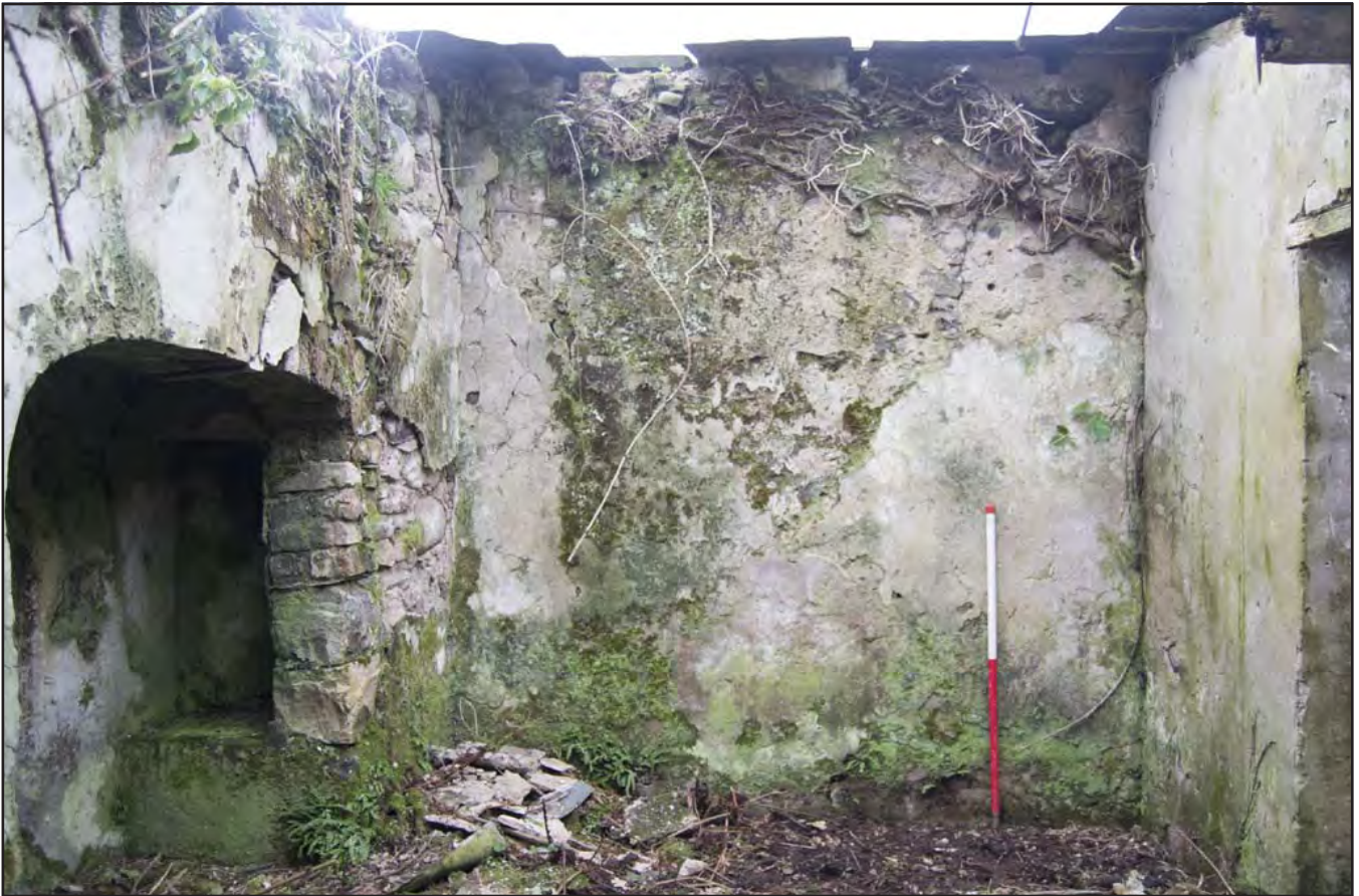
Plate 29: Room 3 - View of Room 3 showing collapsed slate tile roof and slate shelf within inglenook fireplace; scale 1m; view from NE (archive reference: G2743_29).
