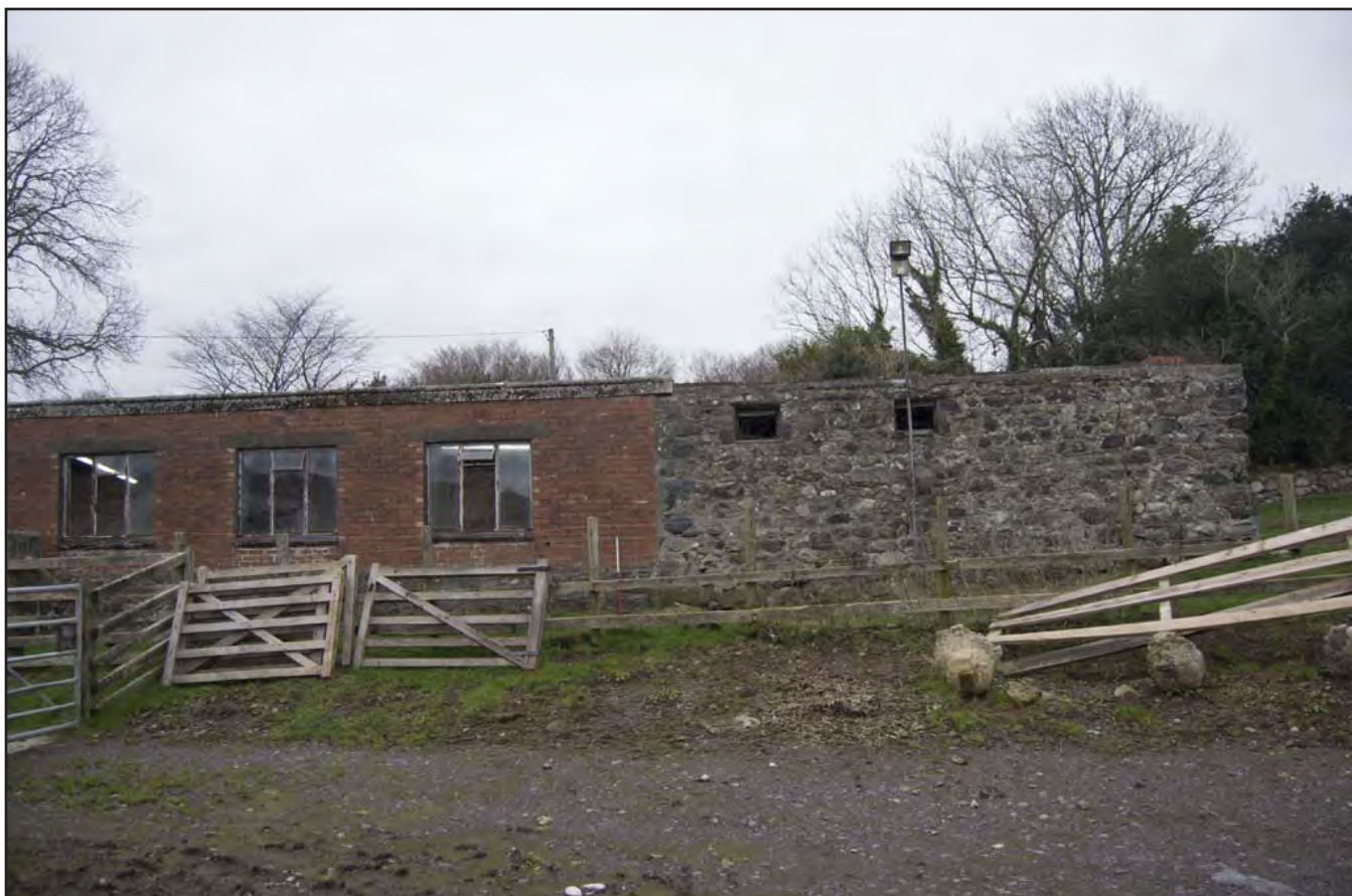
Plate 8: Exterior - SW elevation showing distinct phasing between 19th & 20th century brickwork; scale 1m; view from SW (archive reference: G2743_08).
