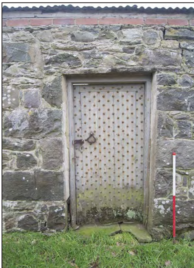
Plate 18: Room 1 - View of reinforced 19th century door - Exterior; scale 1m; view from NE (archive reference: G2743_18).
