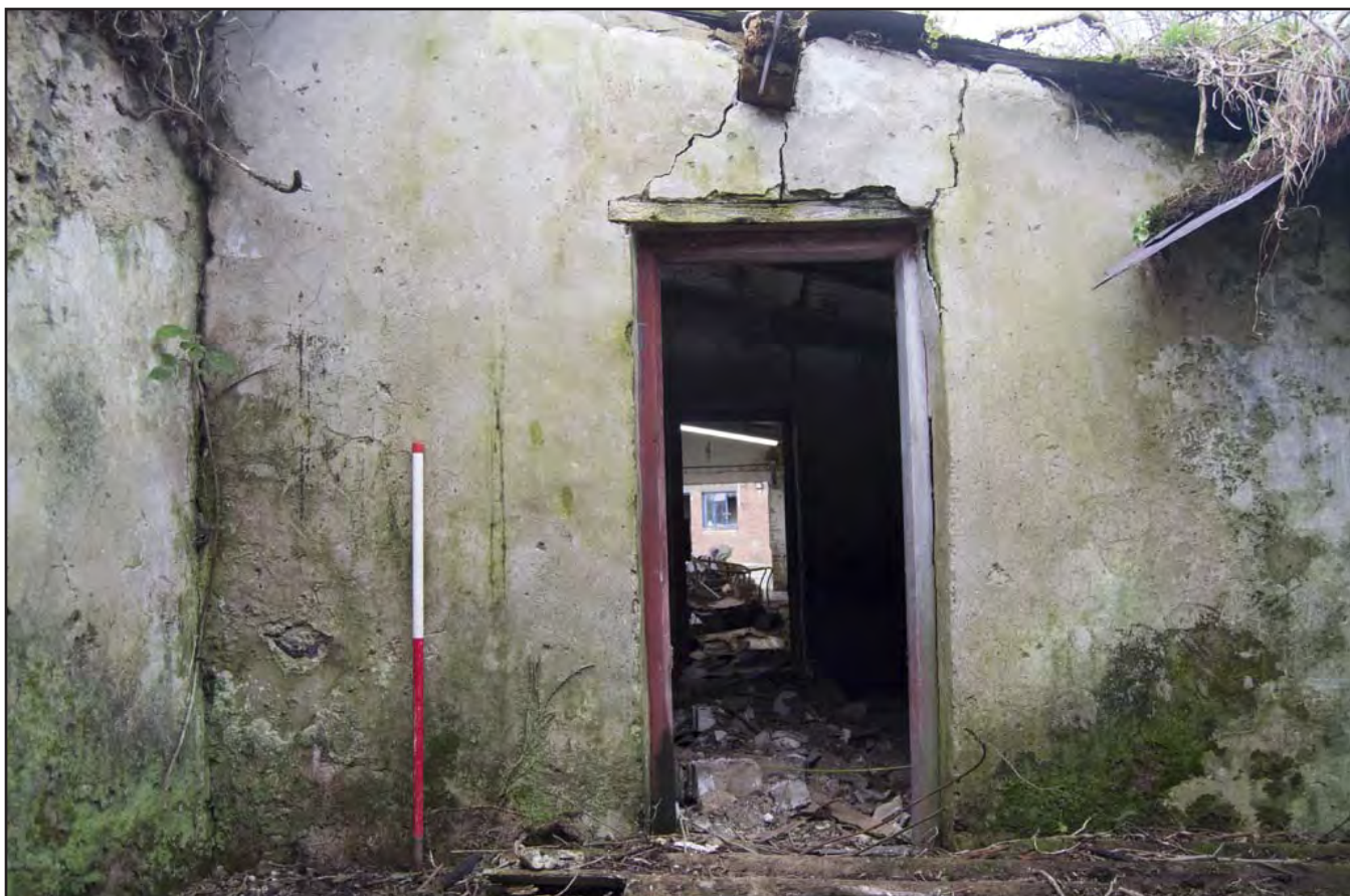
Plate 26: Room 3 - Entrance into Room 3 from Room 2 with lime plaster facing; scale 1m; view from SE (archive reference: G2743_26).
