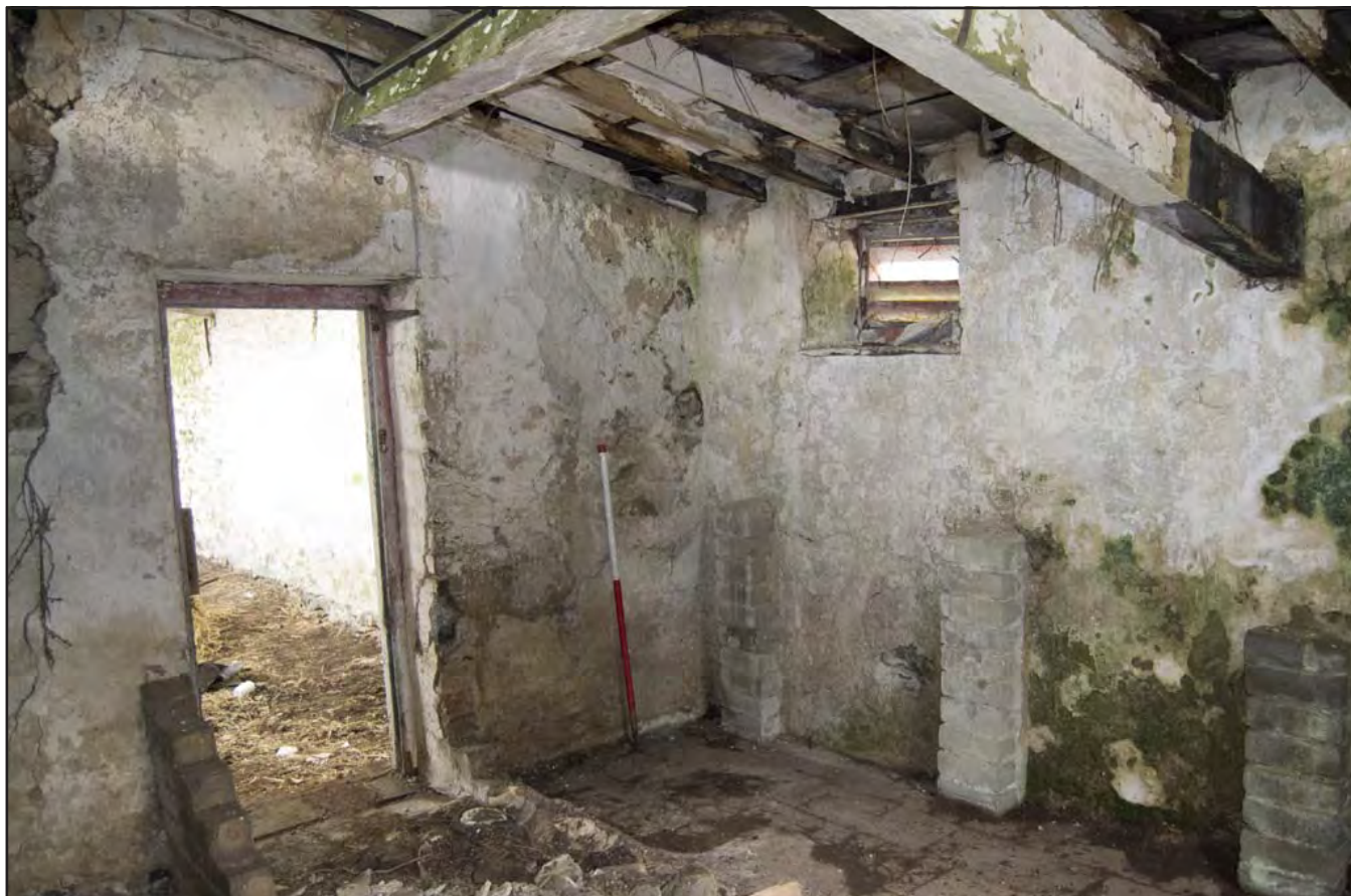
Plate 25: Room 2 - View of NW end of Room 2 with brick dividers and stone tiled floor; scale 1m; view from S (archive reference: G2743_25).
