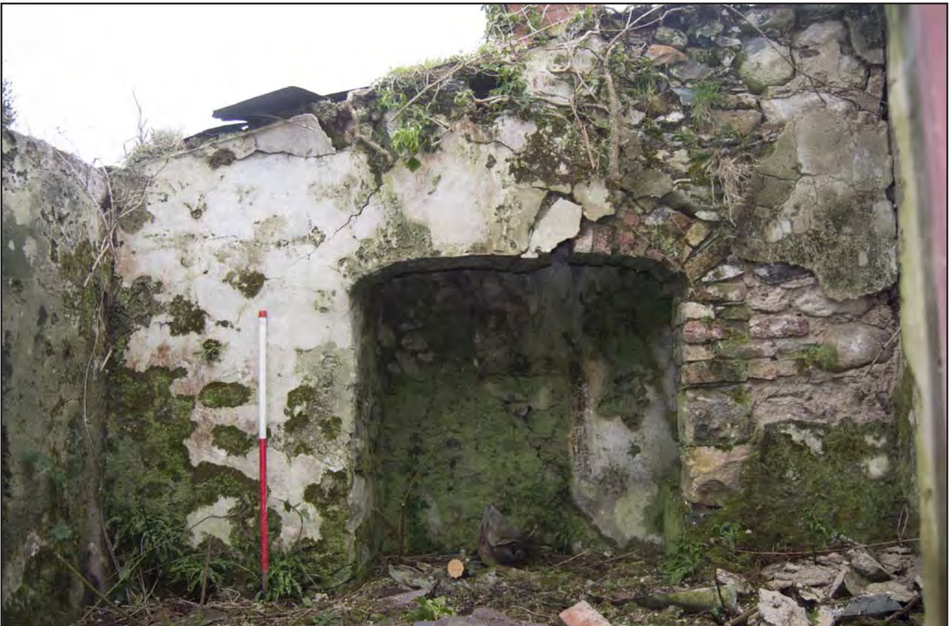
Plate 28: Room 3 - View of voussoir brick inglenook fireplace SE end of Room 3; scale 1m; view from NW (archive reference: G2743_28).
