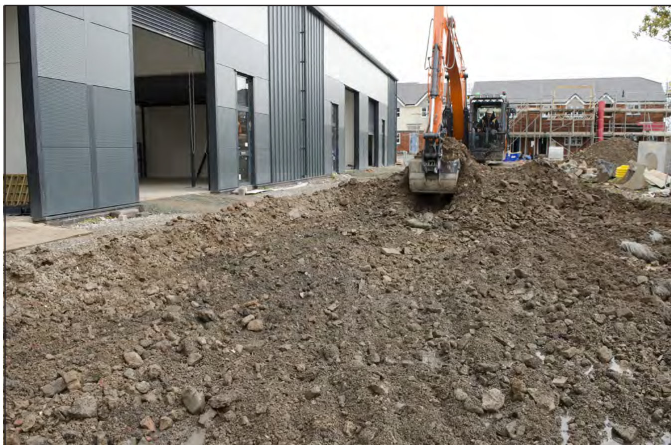
Plate 14: Removal of hardcore for site road adjacent to industrial units; scale not used; view from southwest (archive reference: G2392_363).
