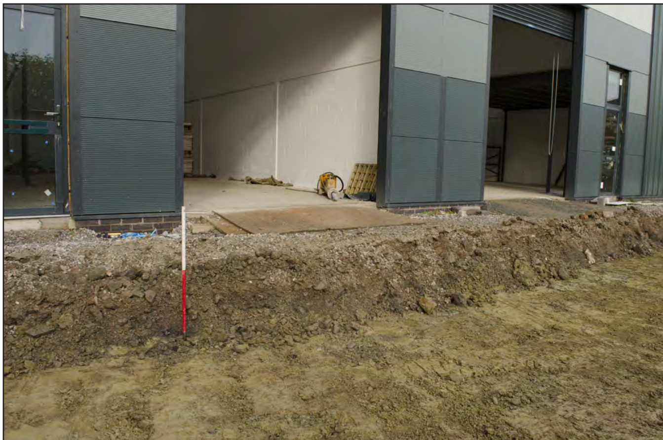
Plate 15: Depth of hardcore for site road; scale 1x1m; view from south southwest (archive reference: G2392_365).
