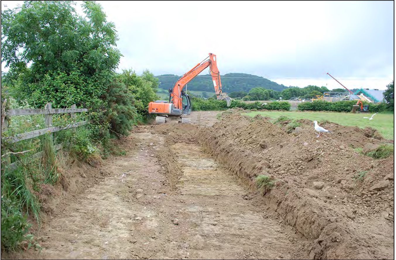
Plate 03: Topsoil strip completed; ; scale not used; view from northwest (archive reference: G2392_304).
