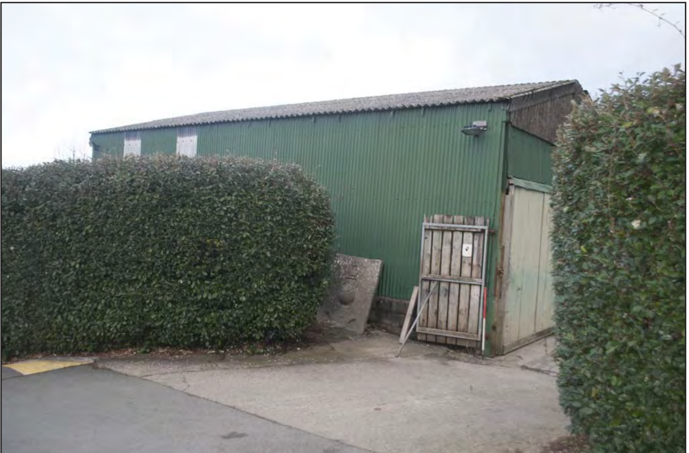
Plate 22: Possible wartime corrugated iron shed with asbestos roof, adjacent to the NE side of the entrance of lot, now used as works yard; scale 1m; view from S (archive reference: G2760_22).
