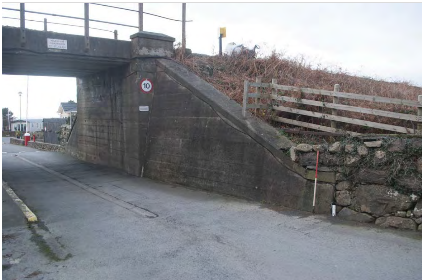
Plate 3: Angled view showing 20th century rendered concrete of NW railway bridge abutment; scale 1m; view from S (archive reference: G2760_03)..
