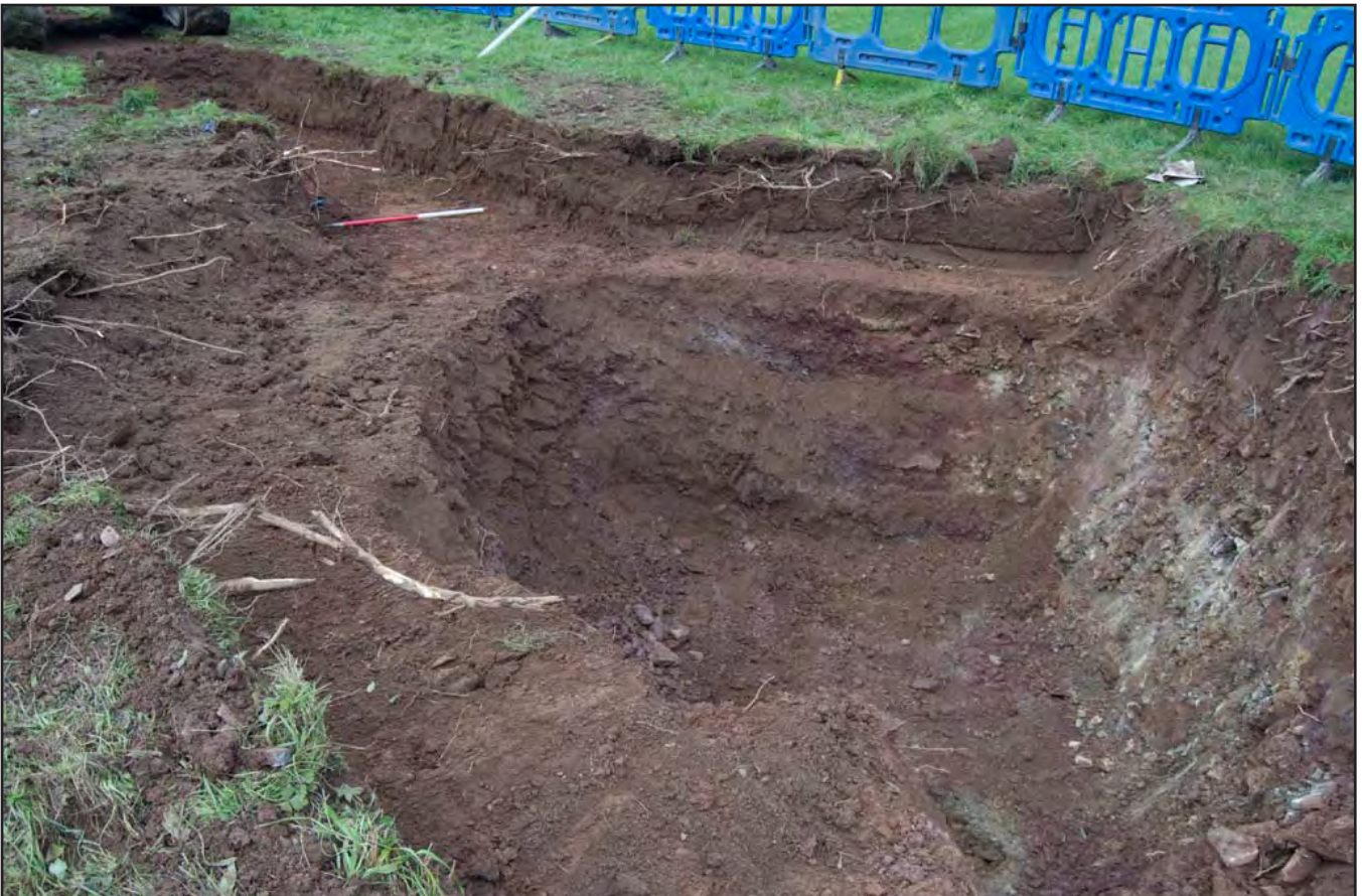
Plate 04: View of chamber area excavated to depth and pipe trench with topsoil and subsoil removed; scale: 1x1m (archive reference: G2751_016).
