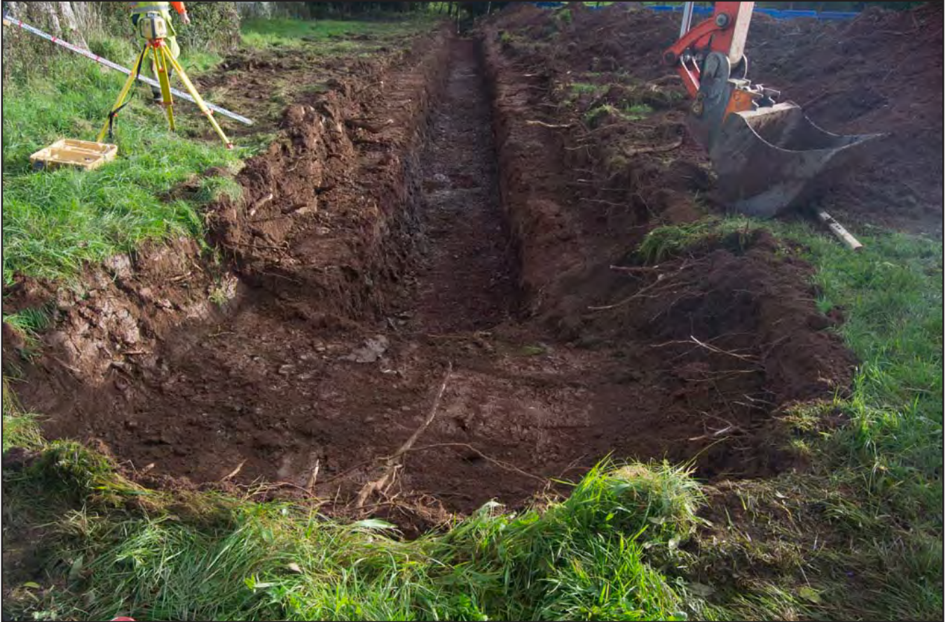
Plate 03: View of the pipe trench and chamber area with topsoil and subsoil removed to the glacial clay; (archive reference: G2751_014).
