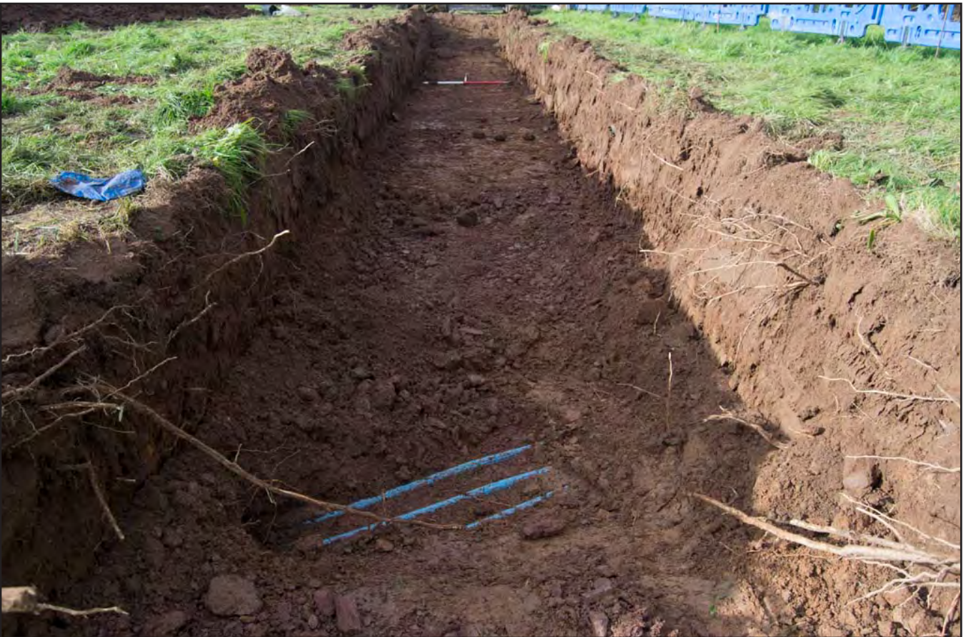
Plate 06: View of the pipe trench from the southeast showing water pipes crossing the trench; scale: 2x1m (archive reference: G2751_19).
