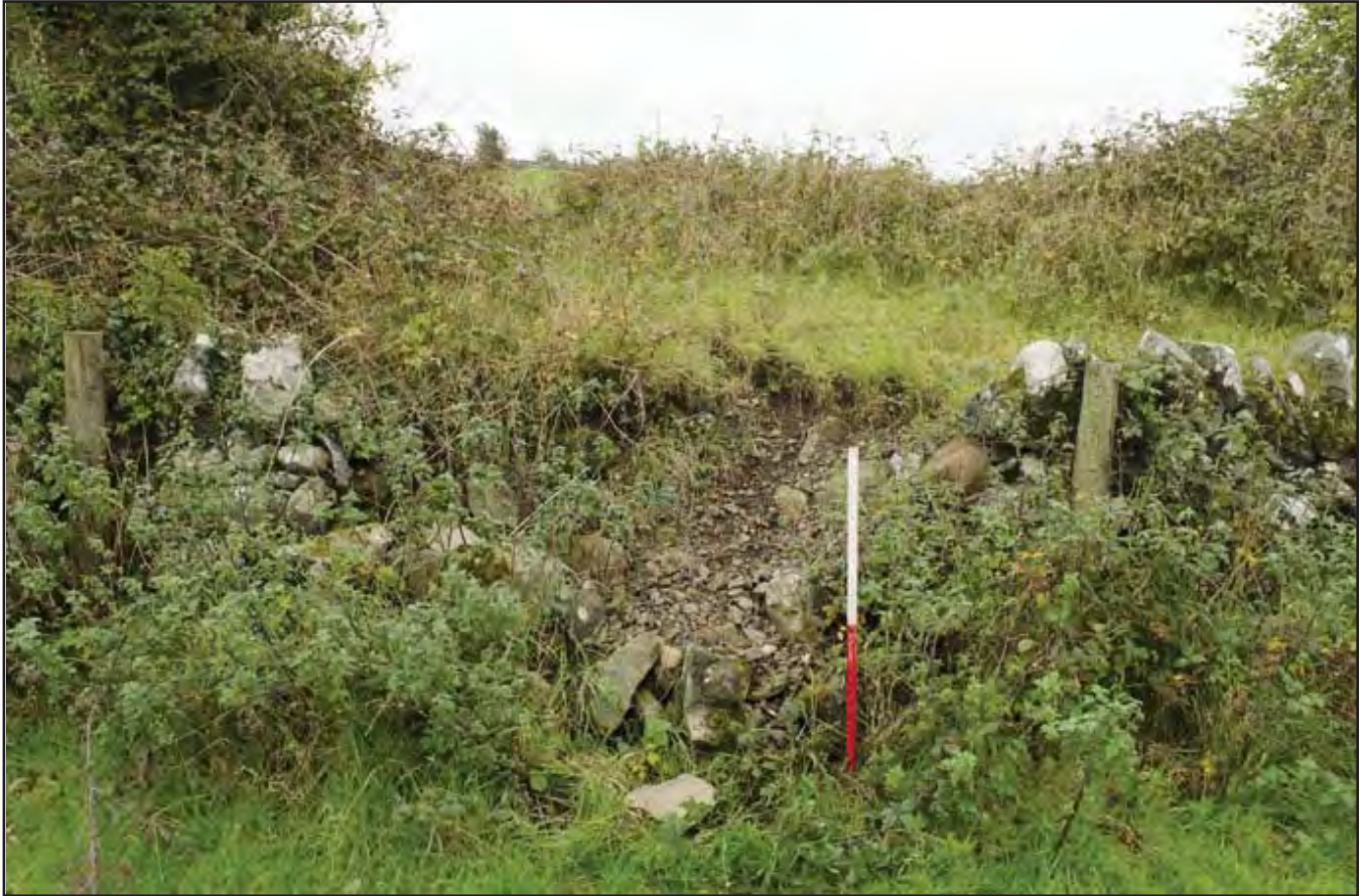
Plate 19: North face of railway embankment, collapsed wall and aggregate (Asset 13); scale 1x1m; view from N (archive reference: G2745_019).
