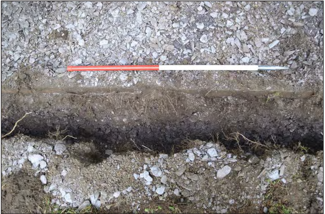
Plate 5: Section of cable trench where it is entirely within the made ground; scale 1m; view from SE (archive reference: G2741_04).
