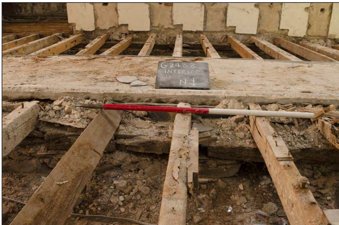
Plate 11: Exposed planks of wood and sleeper wall beneath central aisle; scale: 1x1m (archive reference: G2488_092).
