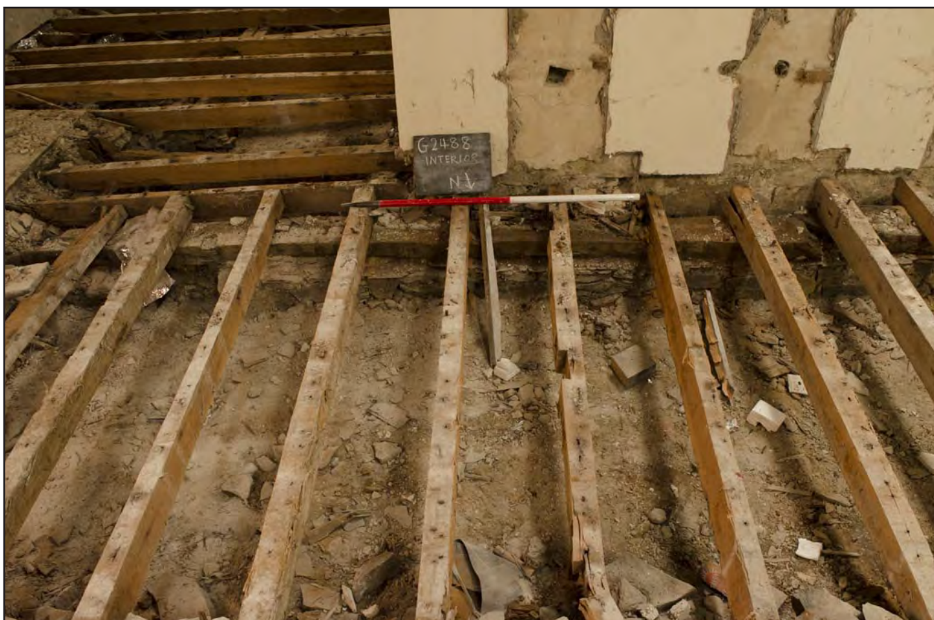
Plate 08: Exposed floor joists, wooden plank and joist hangers along southern wall of church; scale: 1x1m (archive reference: G2488_083).
