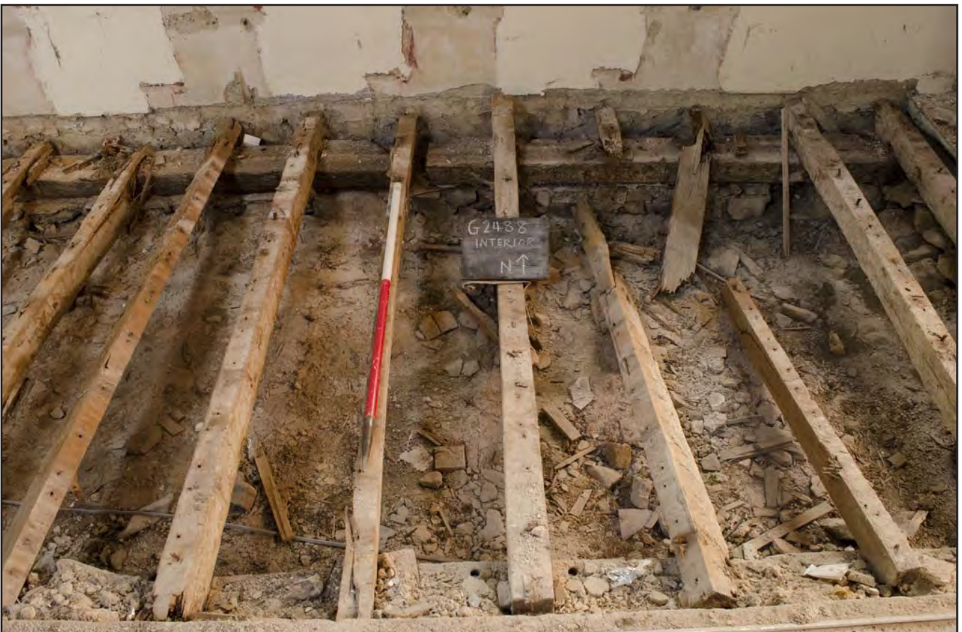
Plate 10: Exposed floor joists along northern wall beneath window; scale: 1x1m (archive reference: G2488_089).
