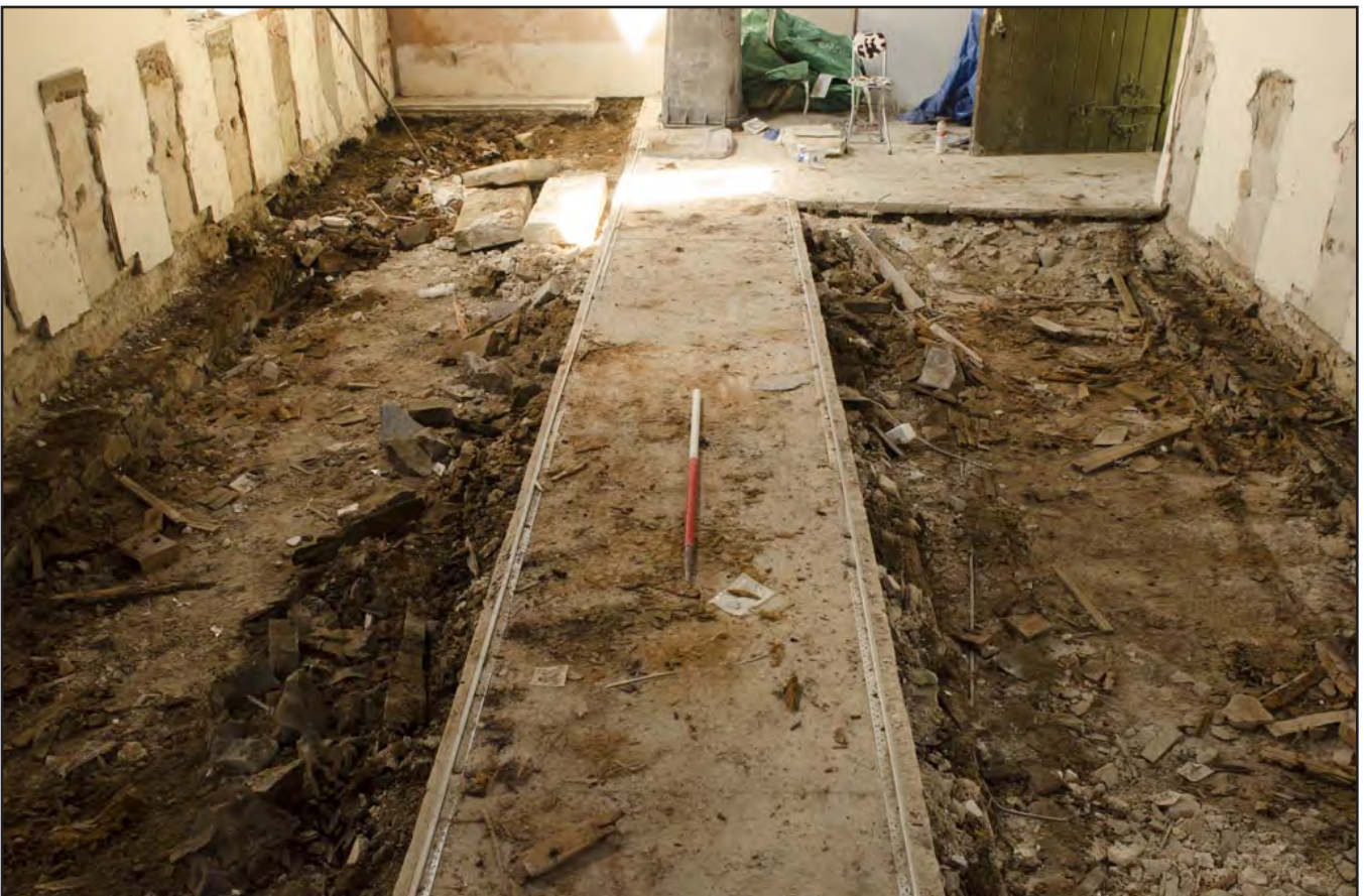
Plate 14: Interior of church after floorboards and joists removed; scale: 1x1m (archive reference: G2488_112).
