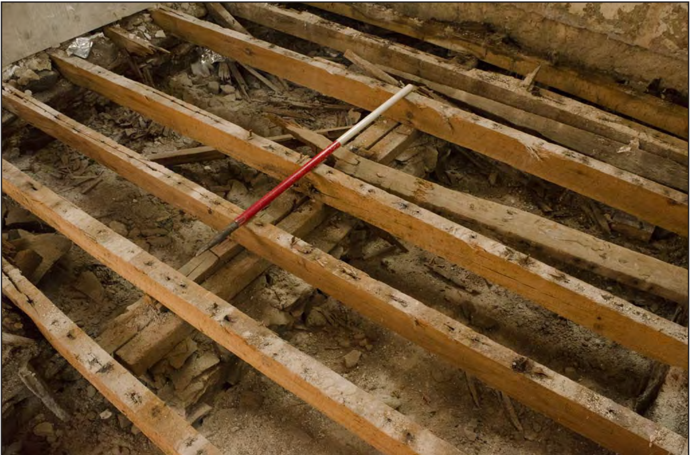
Plate 13: Oblique of central sleeper wall in south wing of church; scale: 1x1m (archive reference: G2488_100).
