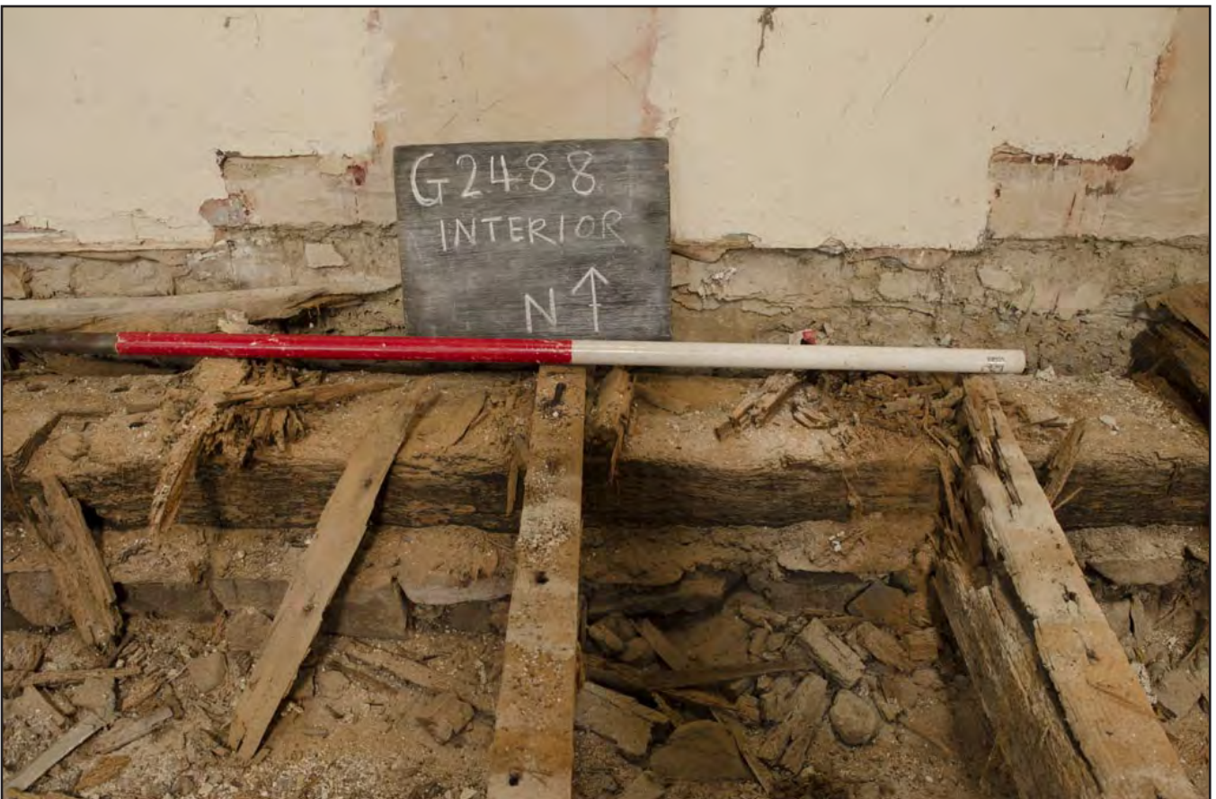
Plate 06: Close-up of elevation of joist hangers and plank along northern wall of church; scale: 1x1m (archive reference: G2488_088).
