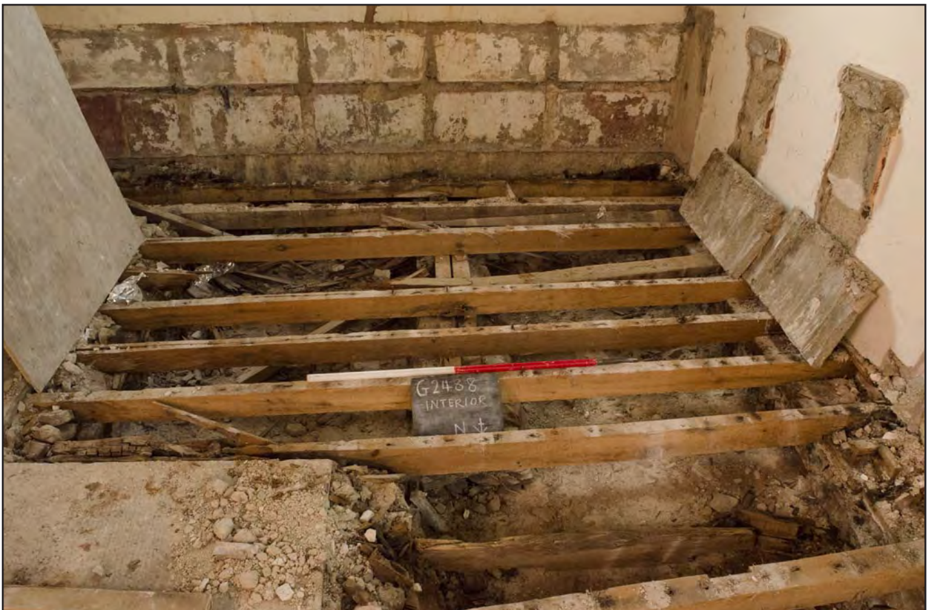
Plate 02: Exposed floor joists in south wing of church; scale: 1x1m (archive reference: G2488_098).
