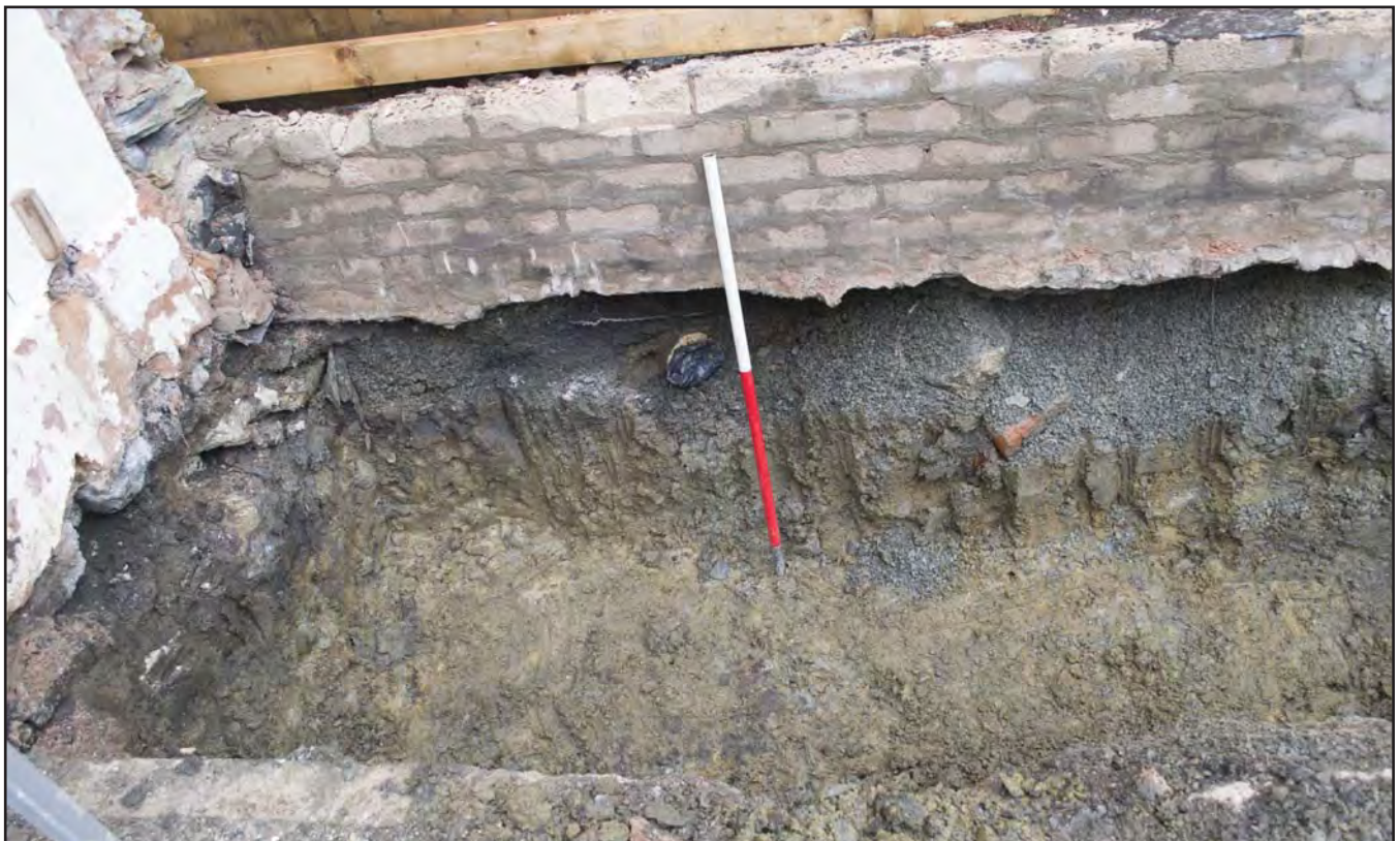
Plate 14: Natural boulder clay visible in foundation trench in south-eastern part of the site; scale: 1m (archive reference: G2738_038)
