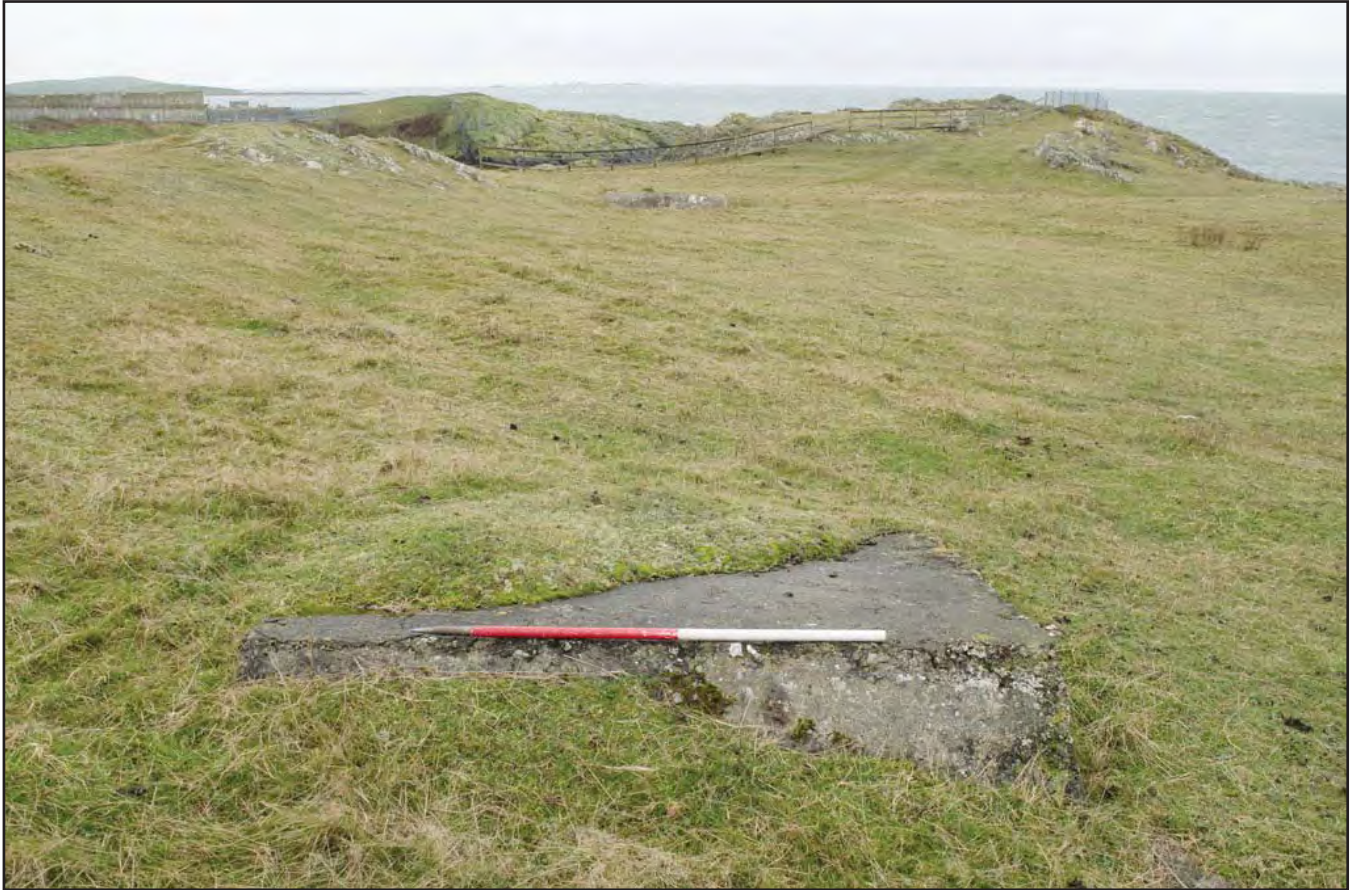
Plate 5: PRN 36598 - Concrete foundations anchor blocks for transmitting masts; scale 1x1m; view from east (archive reference: G2698_020).
