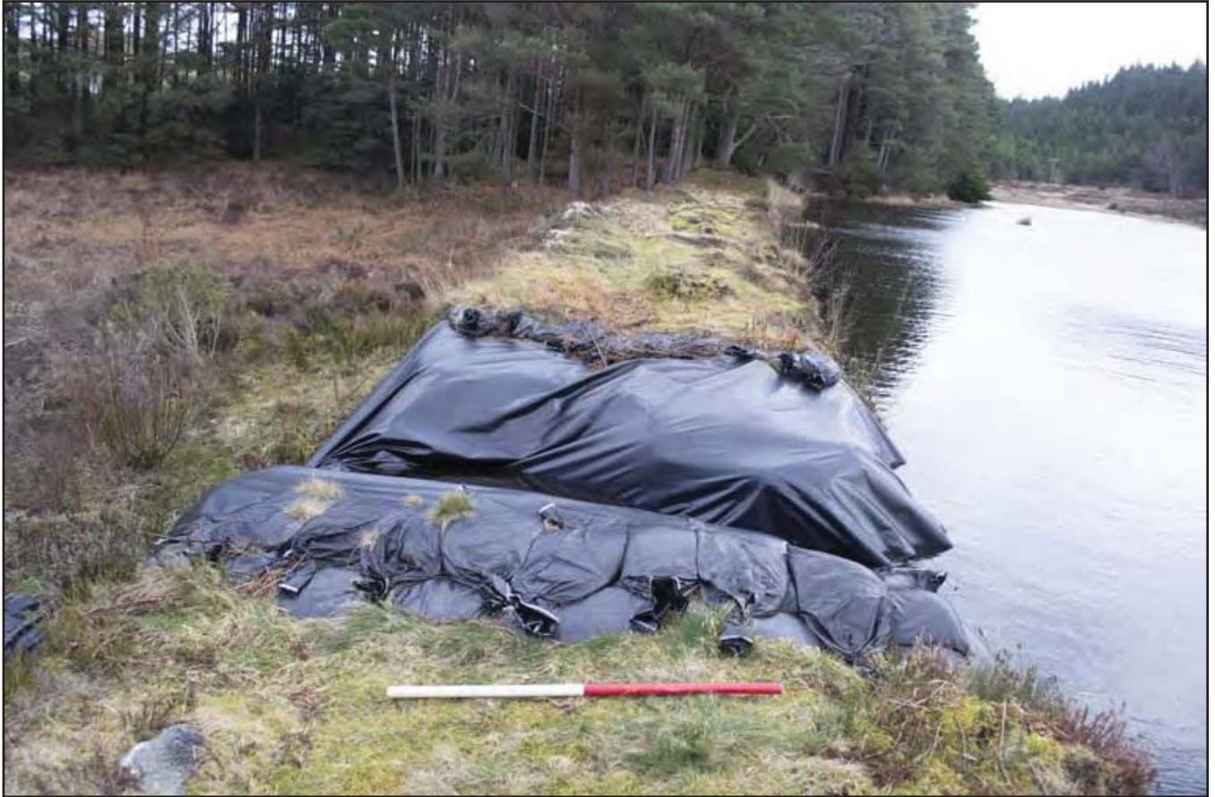
Plate 3: Breach in upper reservoir; scale 1x1m; view from SW (archive reference: G2697_004).
