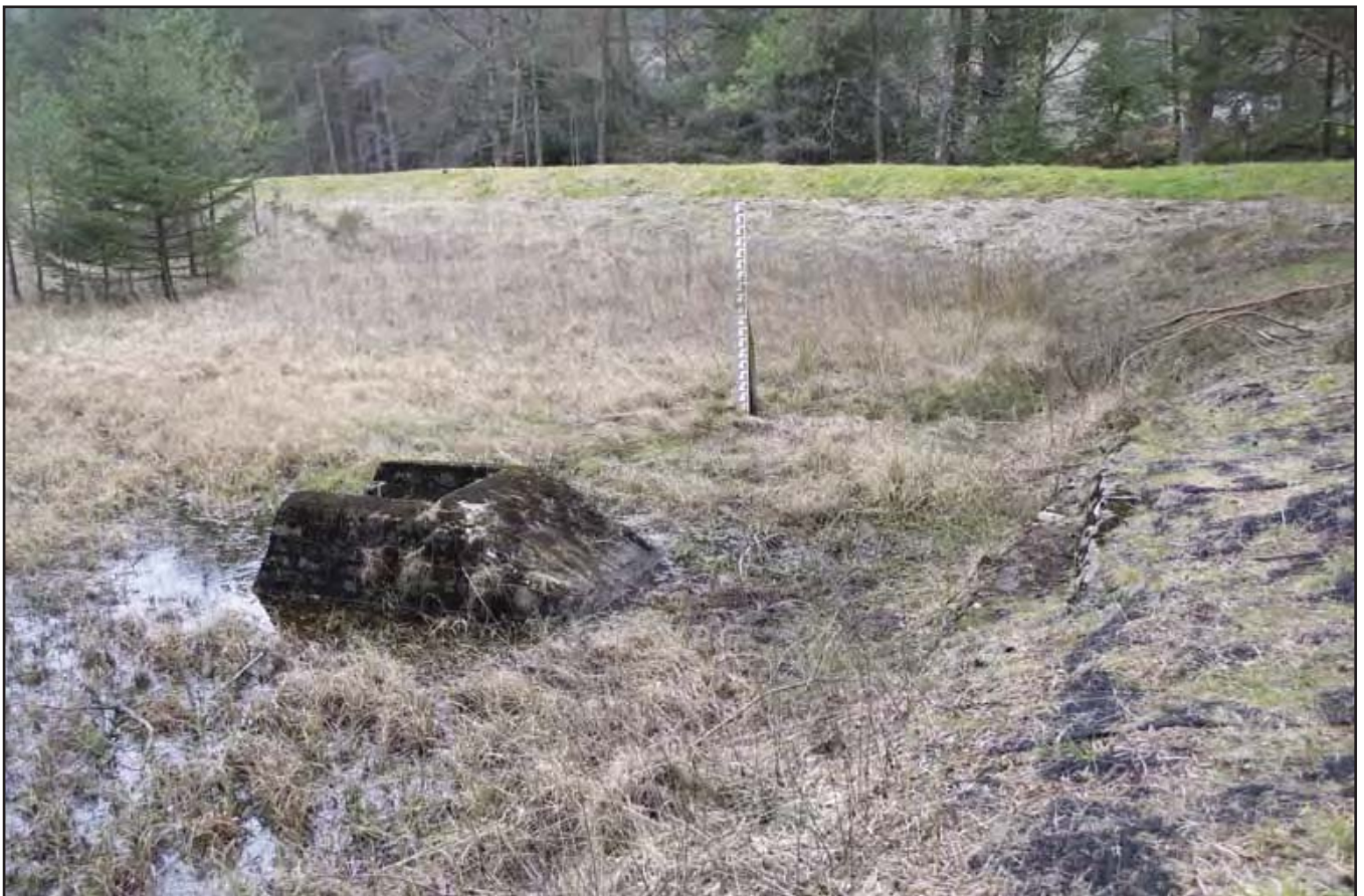
Plate 10: Brick structure for water flow under dam; scale -; view from ESE (archive reference: G2697_026).
