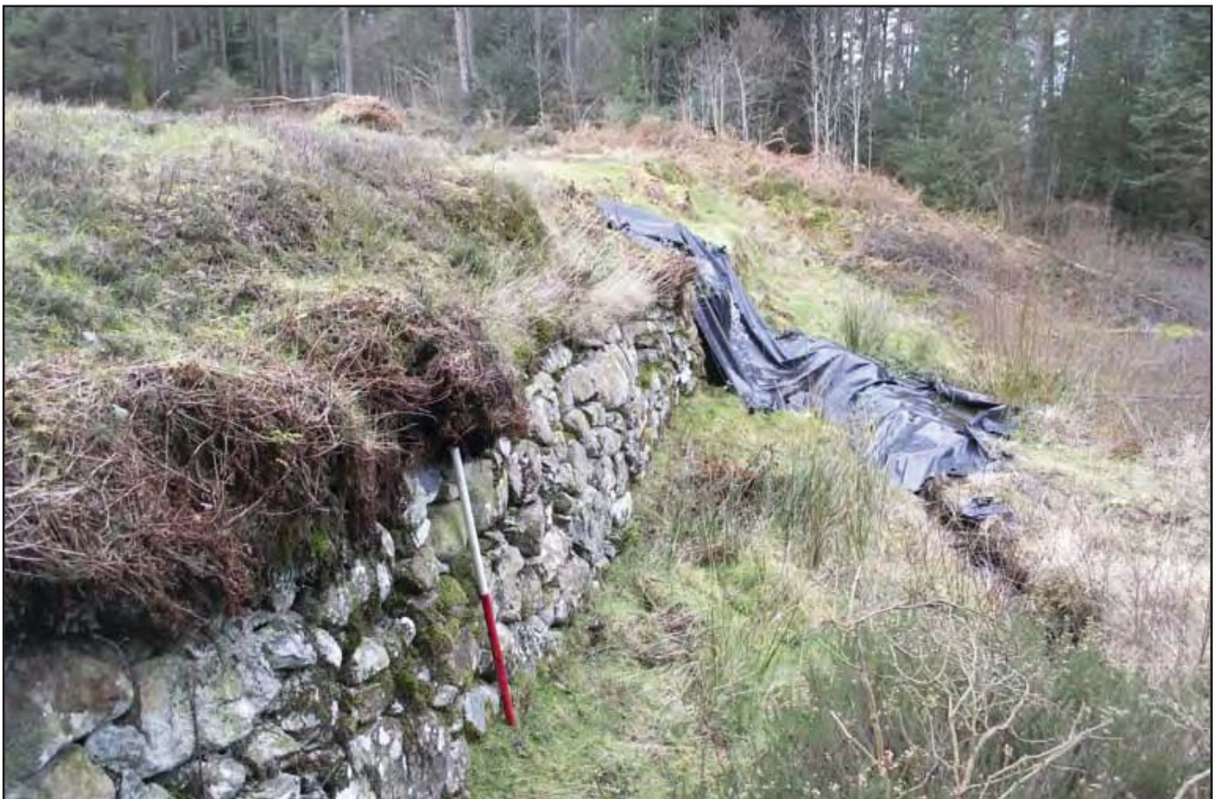
Plate 2: Lower dam revetment; scale 1x1m; view from NNE (archive reference: G2697_013).
