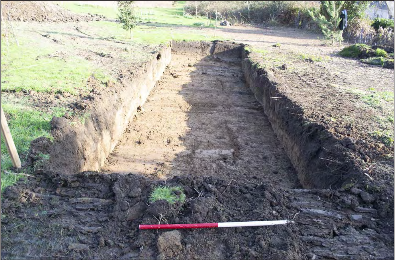
Plate 5: Dig for septic tank and soakaway; scale 1x1m; view from NW (archive reference: G2621_029).
