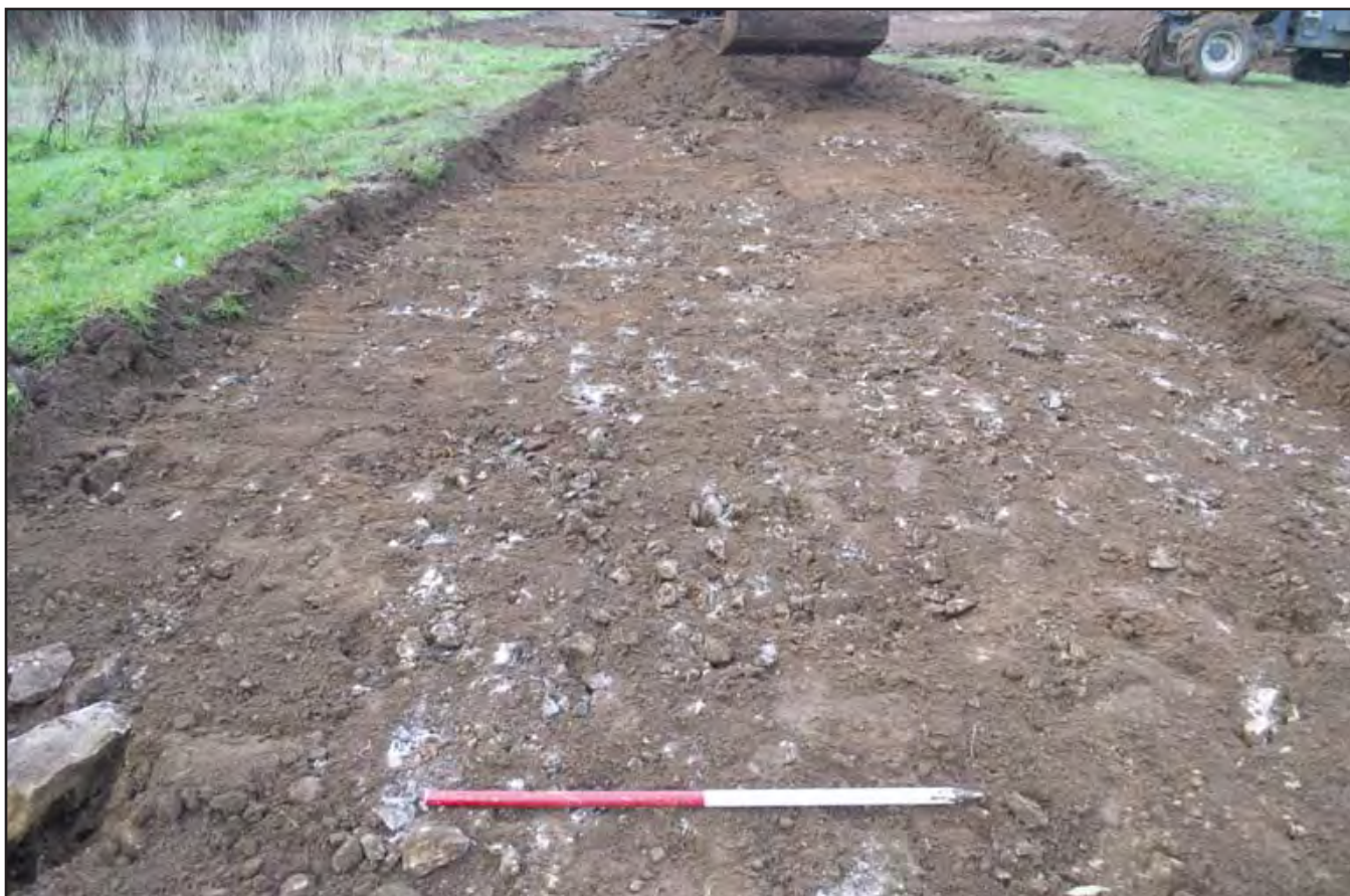
Plate 8: Subsoil strip to formation level - access track; scale 1x1m; view from SE (archive reference: G2666_24).
