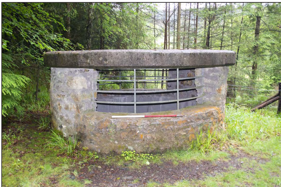
Plate 18: Cover for shaft - Near to Parc Mine Office; scale 1x1m; view from SE (archive reference: G2673_026).
