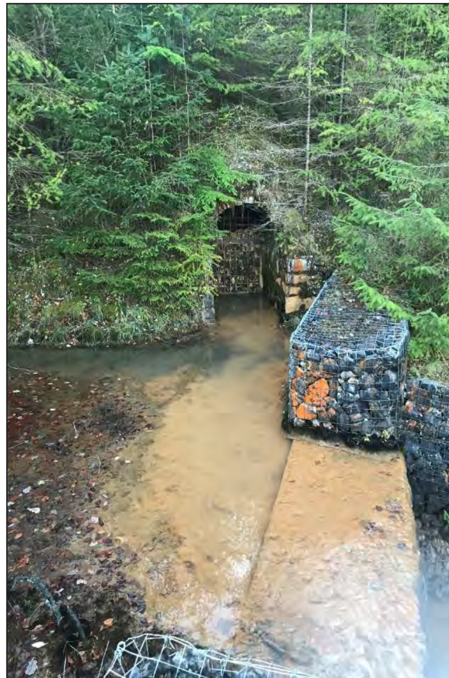
Plate 10: View of adit No:4 portal and gabion basket cascade (The Coal Authority)
