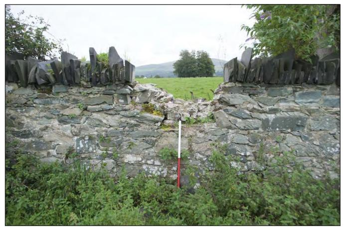
Plate 17: View of damage to Penrhyn Park boundary wall; scale 1x1m; view from W (archive reference: G2663\_025).
