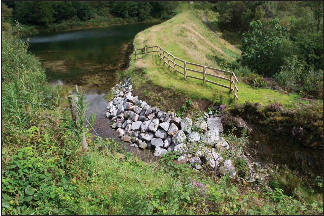
Plate 12: Feature 12: PRN 9146, view of modern revetment works to the Upper Hendre Reservoir dam; scale not used; view from southwest (archive reference: G2660_033).
