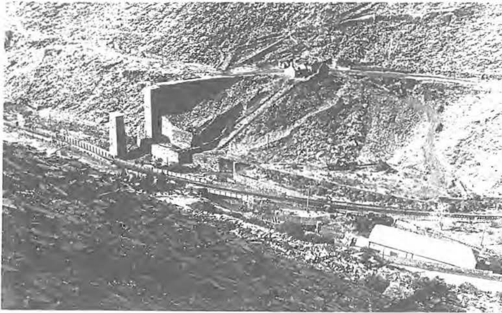
The Llechwedd power house is visible in the bottom right of this photograph, which shows the remains of the Welsh Slate Company's viaduct. This gave access to a tip and a mill area on the far side, which were removed for hardcore in the 1970s. Underneath it ran the Festiniog Railway, joined from 1879 by the LNWR's Blaenau branch, still operational.
