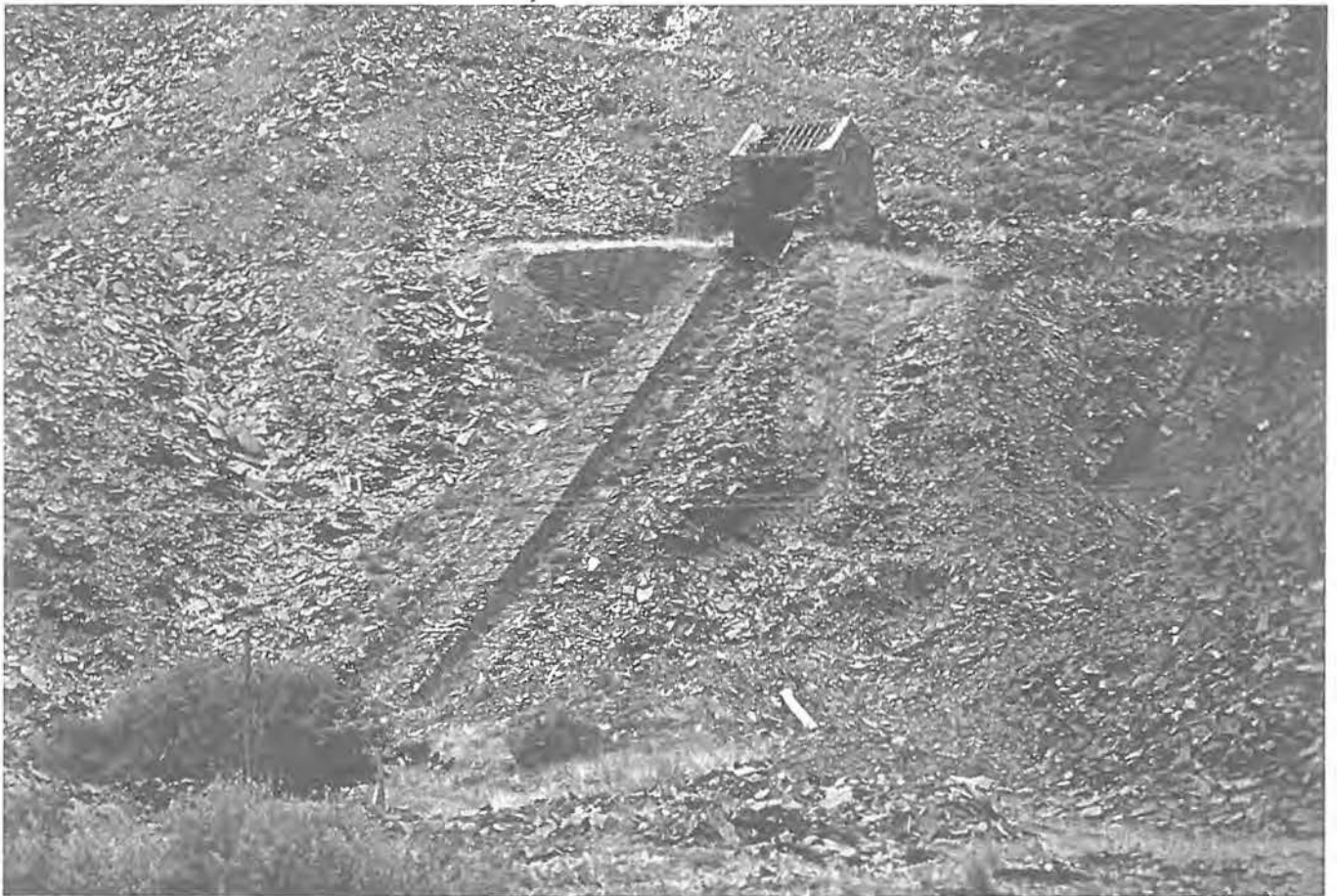
Another method of hauling rock to a higher level was the powered incline. This example at Aberllefenni used the weight of a rail-mounted water-tank to draw the loads upwards on a parallel track.
