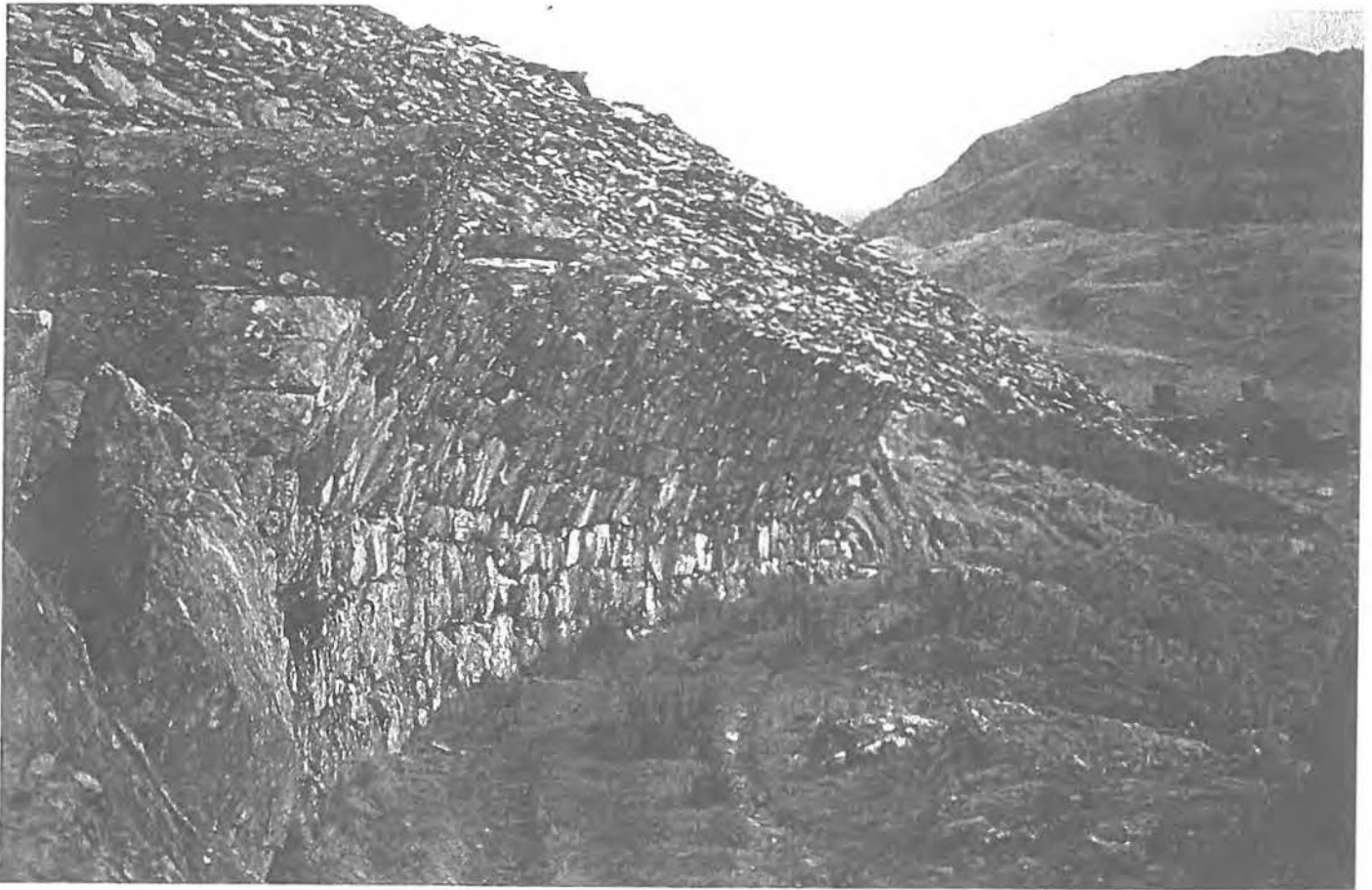
Some quarries built their own transport links to the sea. This shows the route of the 3' gauge Gorseddau railway to Portmadoc, running alongside the quarry's distinctive retaining wall.
