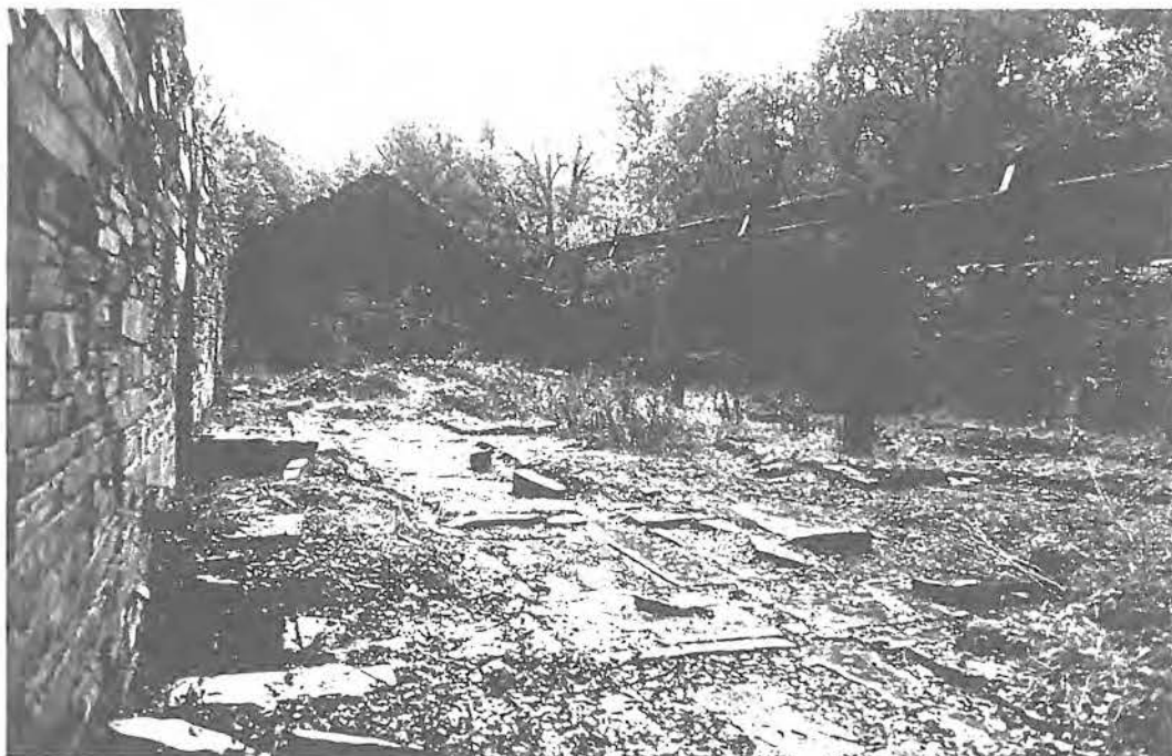
Hafodlas quarry was extensively mechanised in the 1860s. The gantry crane survives, and bases for the Hunter patent saw are visible.
