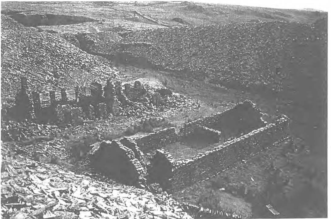
The remoteness of many of the sites obliged managers to build accommodation for their men. This building, the quarrymen's barracks at Glanrafon quarry near Rhyd Ddu, is the only known Gwynedd example of a dual row, a building constructed against a hillside in which entrance to the ground floor was at one side and to the first floor at the other.
