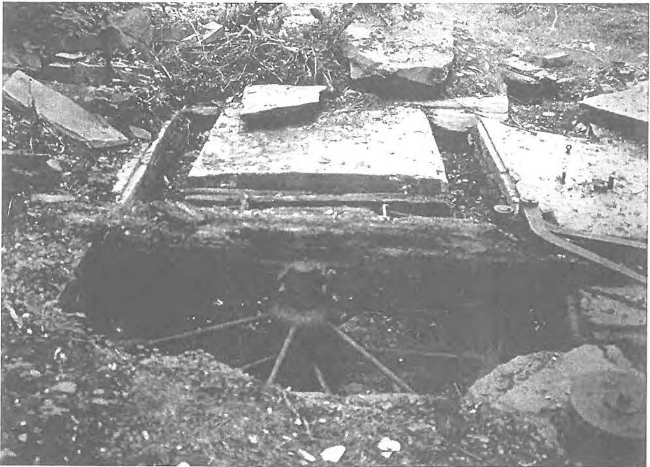
At the incline summit the rope was passed either round a drum on a horizontal axis, or, as here at Hafodlas quarry, Betws y Coed, a sheave.
