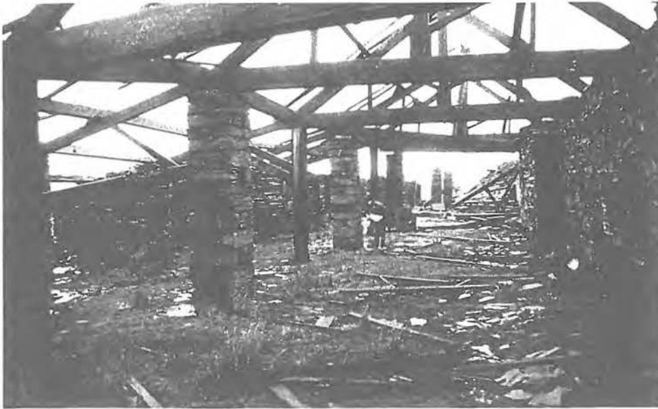
Rhos quarry's mill is a blend of the old and the new. The larger trusses cover a machine area, but to the left are the traditional shelters where individual quarrymen split the slates.
