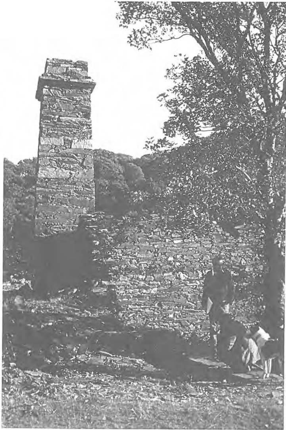
Steam-powered haulage shafts on the lines of a colliery were rare in Gwynedd slate quarries. Nevertheless, the remains of such a system survive at Ty Mawr East in Dyffryn Nantlle.
