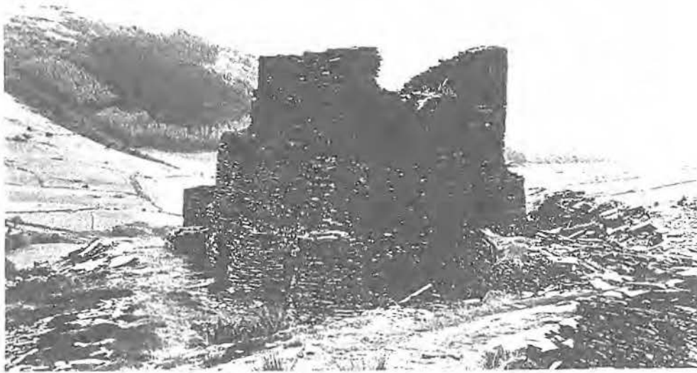
This strongpoint at Cwm Machno quarry supported the summit of a water-balance incline.
