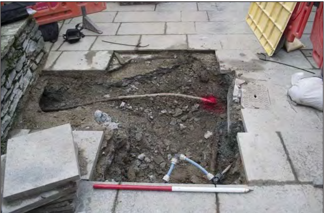
Plate 12: Post-ex shot of trench extension showing exposed services with fault (sprayed red). - Shot from SSW ; scale: 1x1m (archive reference: G2636_012).
