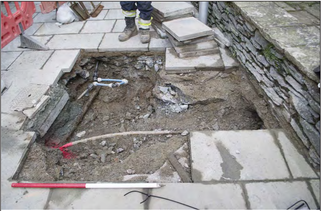
Plate 10: Shot of fully excavated trench extension western side of boundary wall showing mains water, electric and water services. - Shot from SSW; scale: 1x1m (archive reference: G2636_010).
