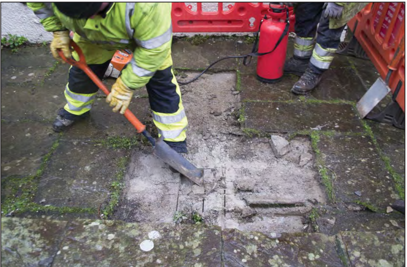
Plate 4: Working shot showing hand removal of flagstones and layer of modern concrete. - Shot from W ; scale: Not used. (archive reference: G2636_004).
