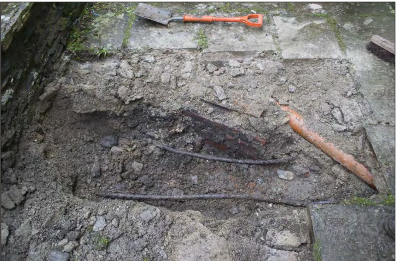
Plate 6: Shot showing x2 exposed cables, manhole and modern ceramic drainage pipes x2.- Shot from SSW ; scale: Not used. (archive reference: G2636_006).
